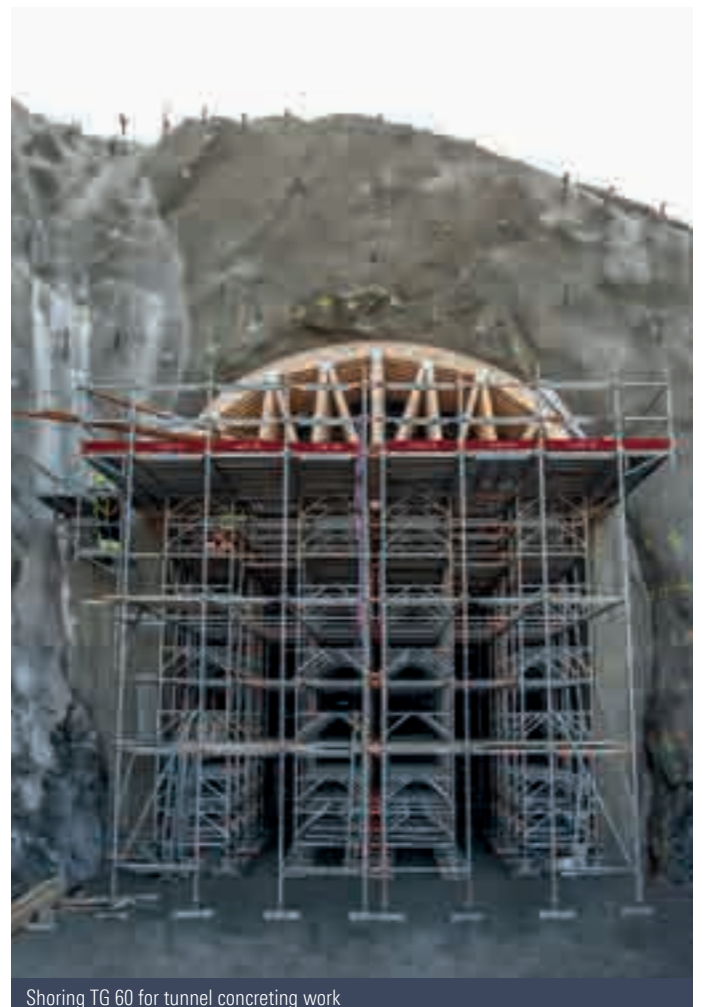
Allround Shoring Frame TG 60 with integrated FW System for vehicle passage opening
