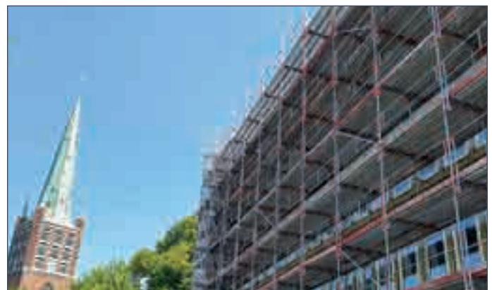
Facade work scaffolding with I-Guardrails
