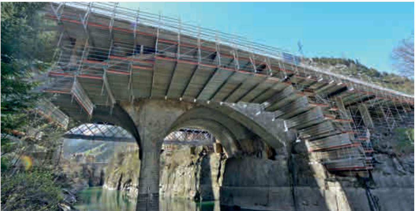
Bridge underside scaffolding with two levels made from Aluminium FlexBeam at a viaduct
