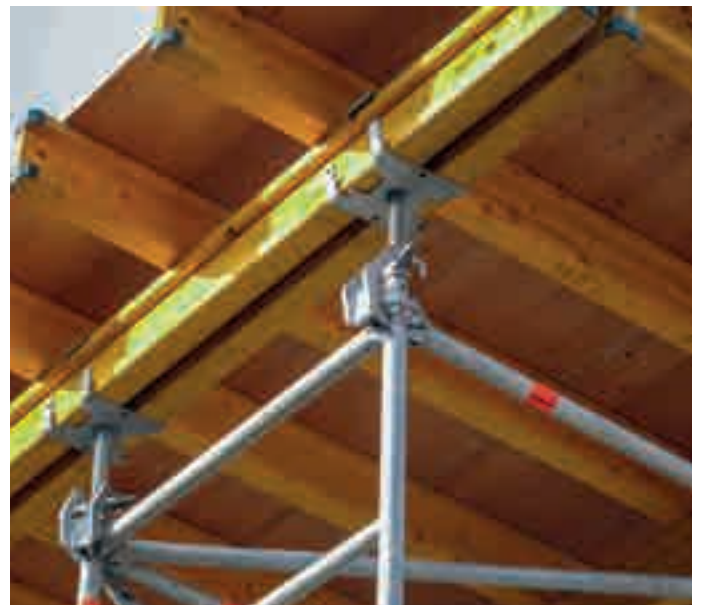
Shoring TG 60 as a slab table with pull-resistant connection of the formwork to the shoring towers
