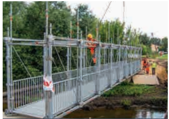
Temporary bridge with approx. 18 metre span
