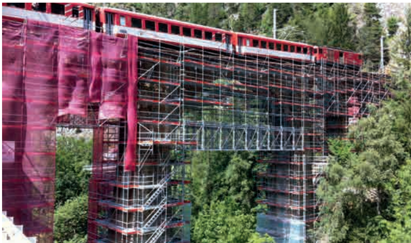
Free-standing work scaffolding on a stone arched bridge with Allround Bridging System for support
