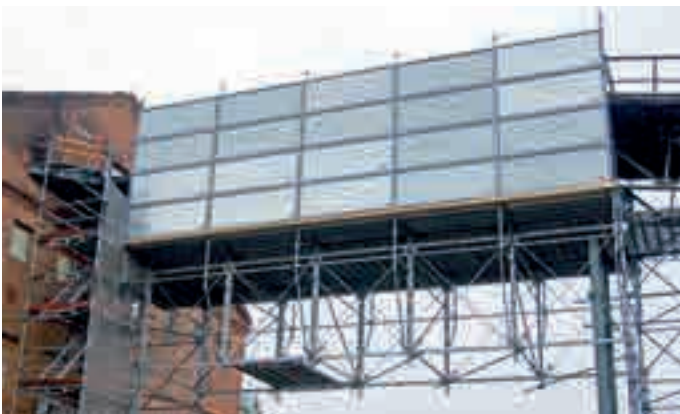
Work scaffolding covered using the Protect System on a pipeline bridge for fire damage repair
