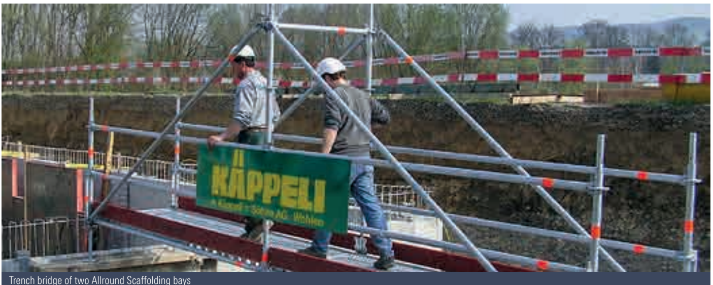
Trench bridge of two Allround Scaffolding bays
