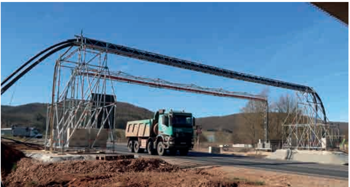
Pipeline bridge using Allround support scaffolding and steel lattice beams
