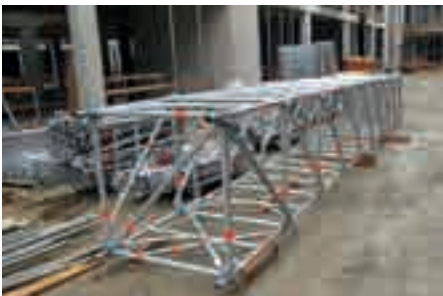
Preassembly of TG 60 Shoring Tower on the ground
