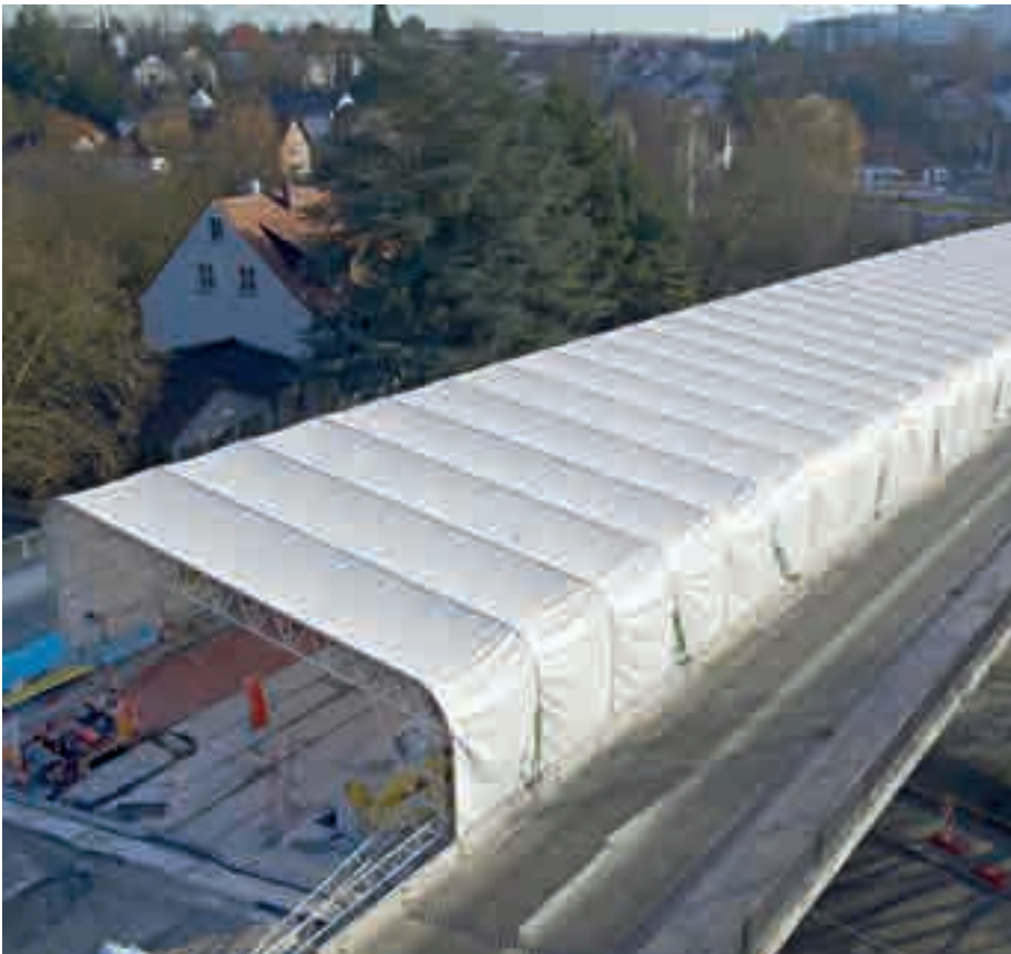
Road surface repair regardless of weather conditions
