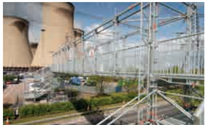
Temporary footbridge using Allround Bridging System with Stairtower 750 to assist site logistics
