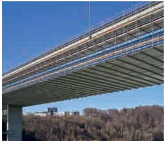
Approx. 7000 m 2 -sized bridge underside scaffolding with FlexBeam at a steel composite bridge
