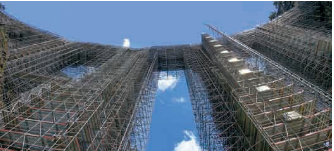
Free-standing work scaffolding on stone arched bridge
