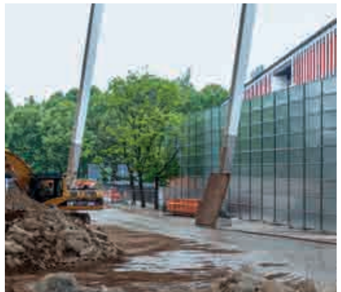
Noise and dust protection wall using Protect System, Mercedes Benz Arena, Stuttgart
