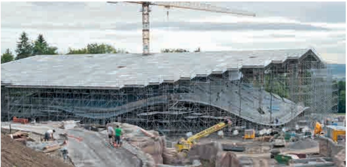
Weather protection roof during construction of an animal enclosure
