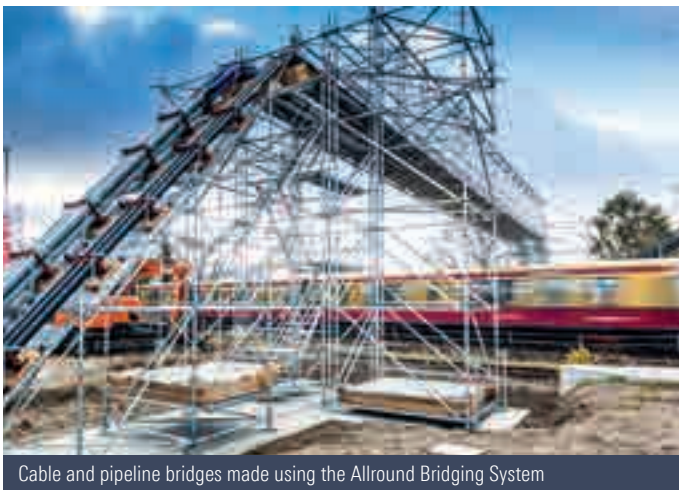
Pipeline bridge using steel trusses
