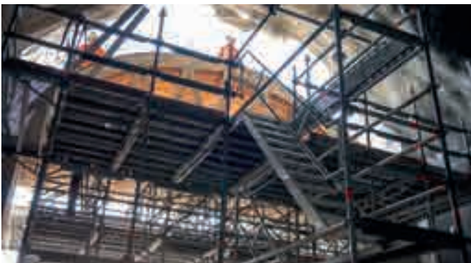
Integration of stair accesses into shoring structures
