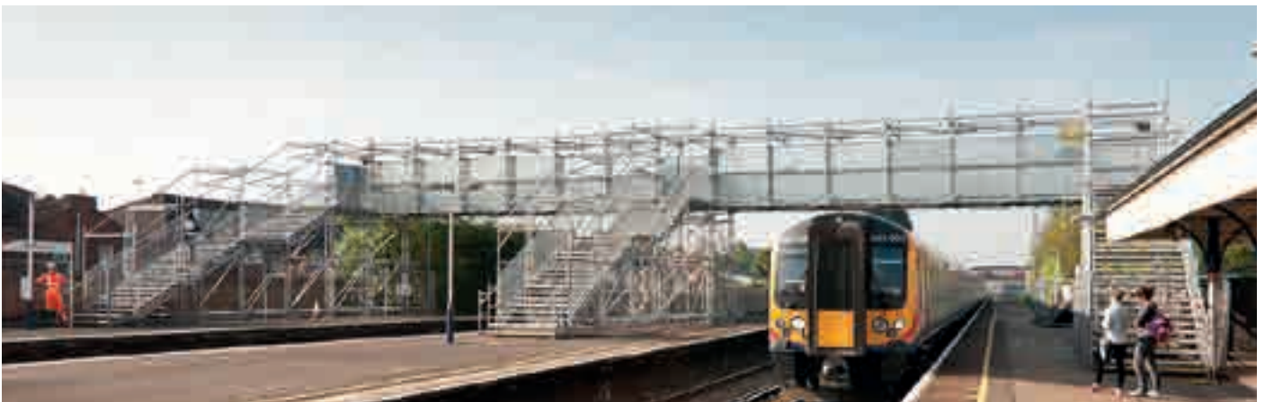
Temporary footbridge using Allround Bridging System on railway platform with Stairtowers 750 and internal Protect enclosure
