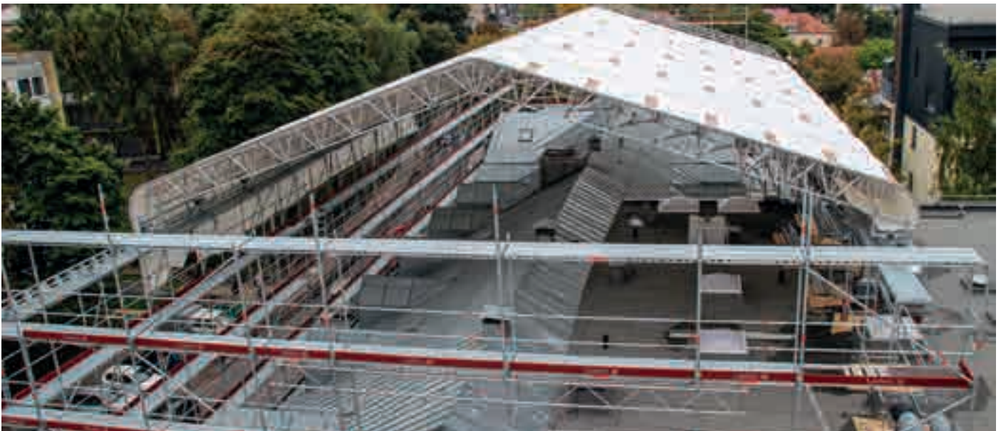
Mobile Keder Roof XL on SpeedyScaf during roof work on an office building
