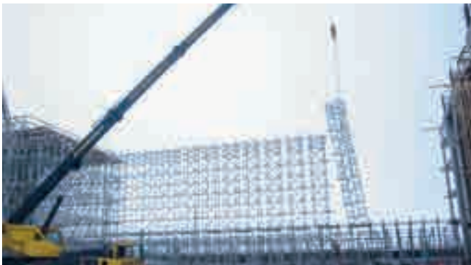
Combination of upright and on-the-ground assembly of individual Shoring Towers TG 60 to save time during assembly
