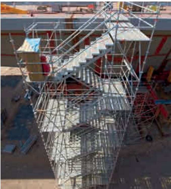
Site stairtower 200 for access to road surface
