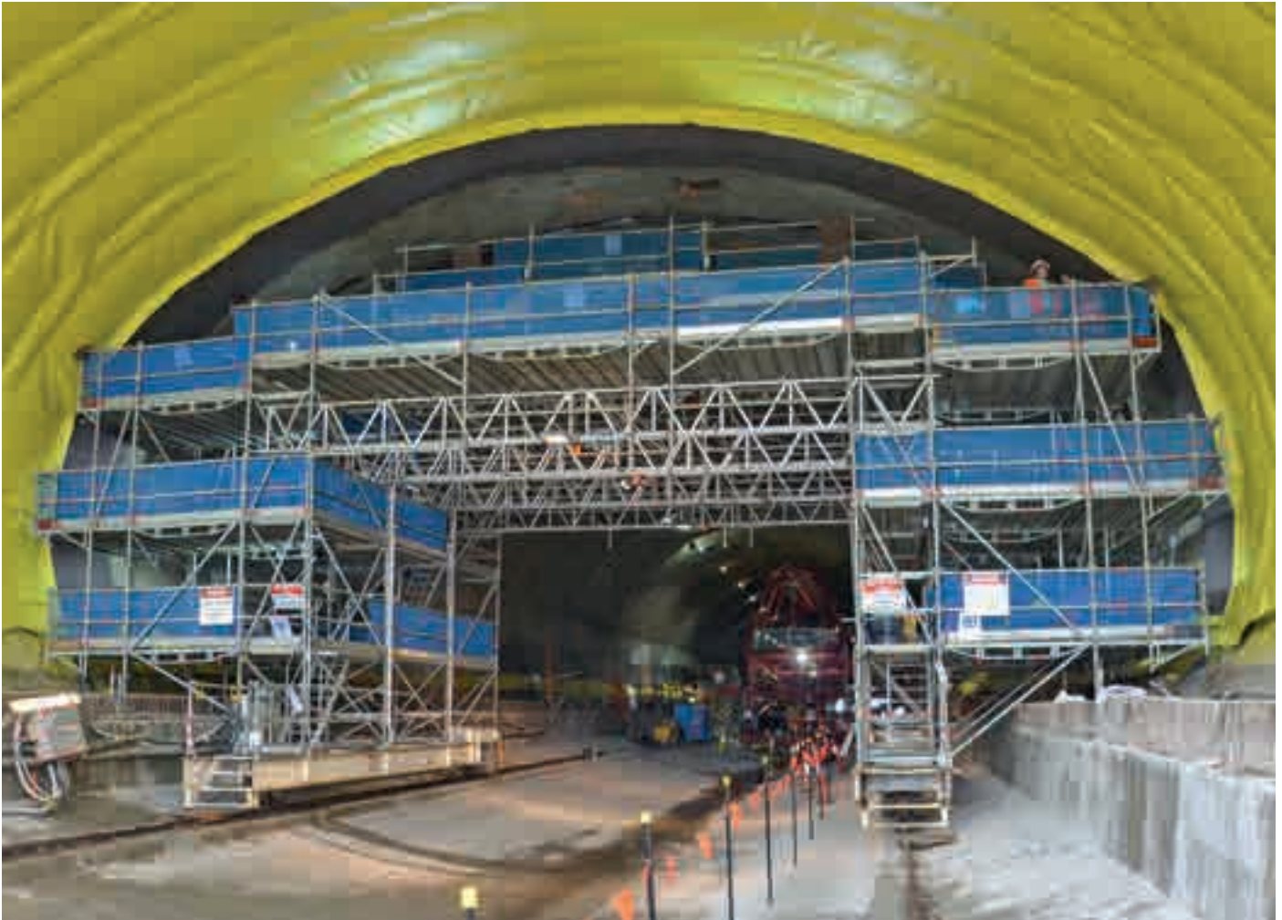
Mobile tunnel scaffolding running on rails
