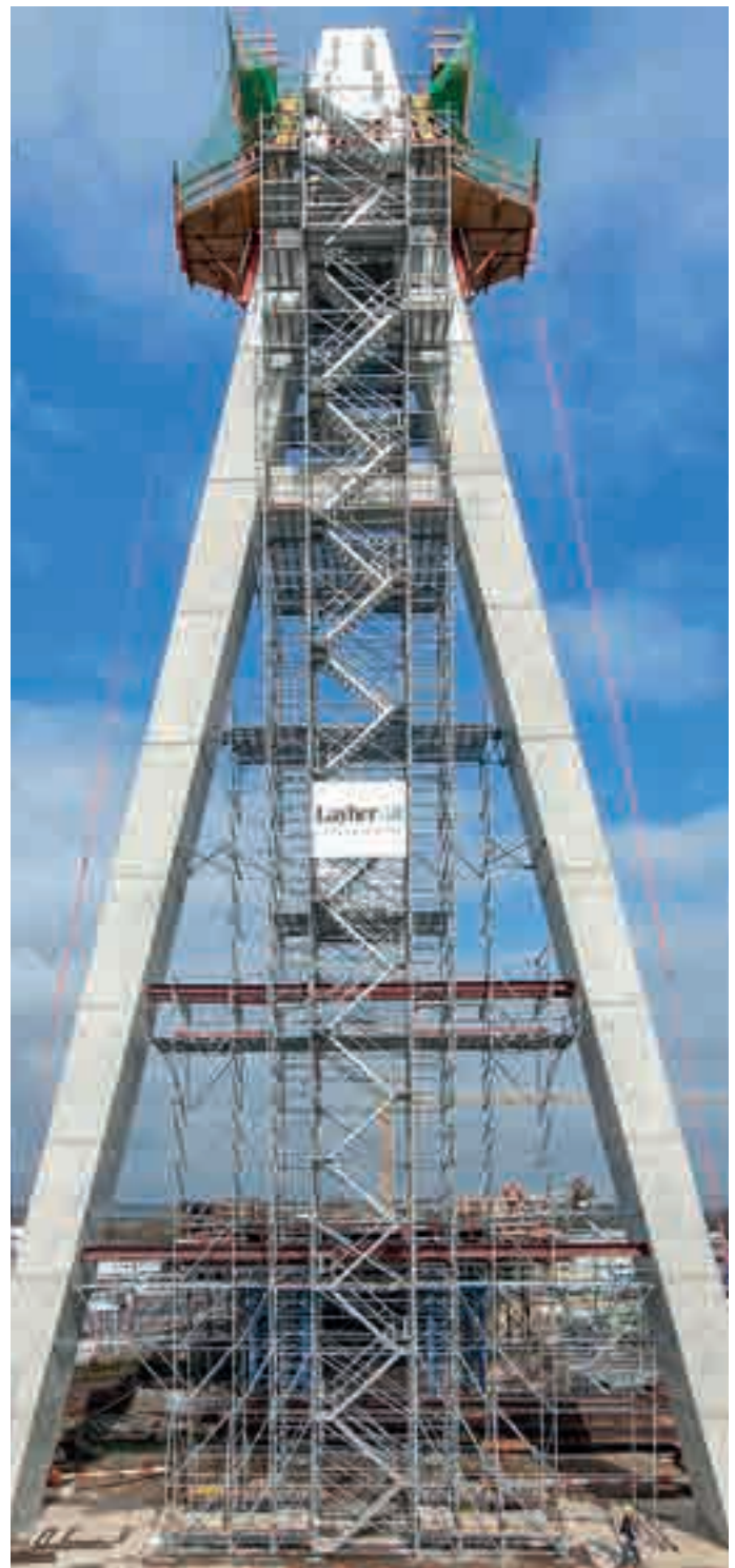
Shoring TG 60 and platform stairtower at the pylon of a cable-stayed bridge
