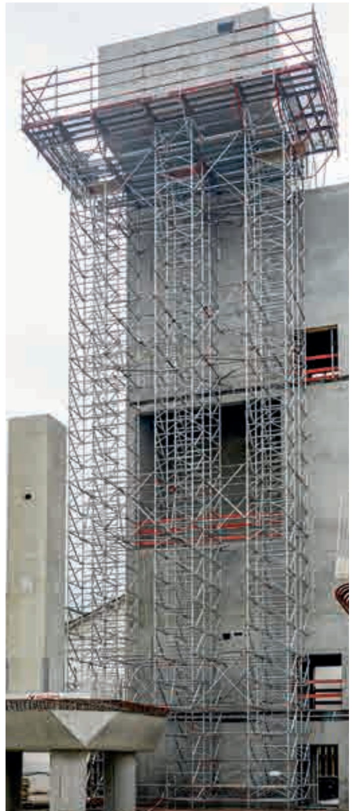
High support towers made from Allround Shoring TG 60 with system-integrated bracket-mounted walkways
