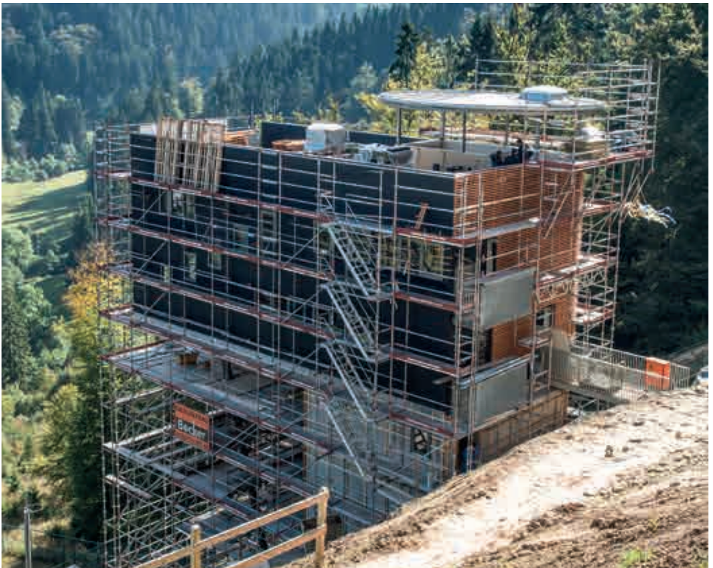
Allround work scaffolding in a complex terrain geometry, with integrated stair access
