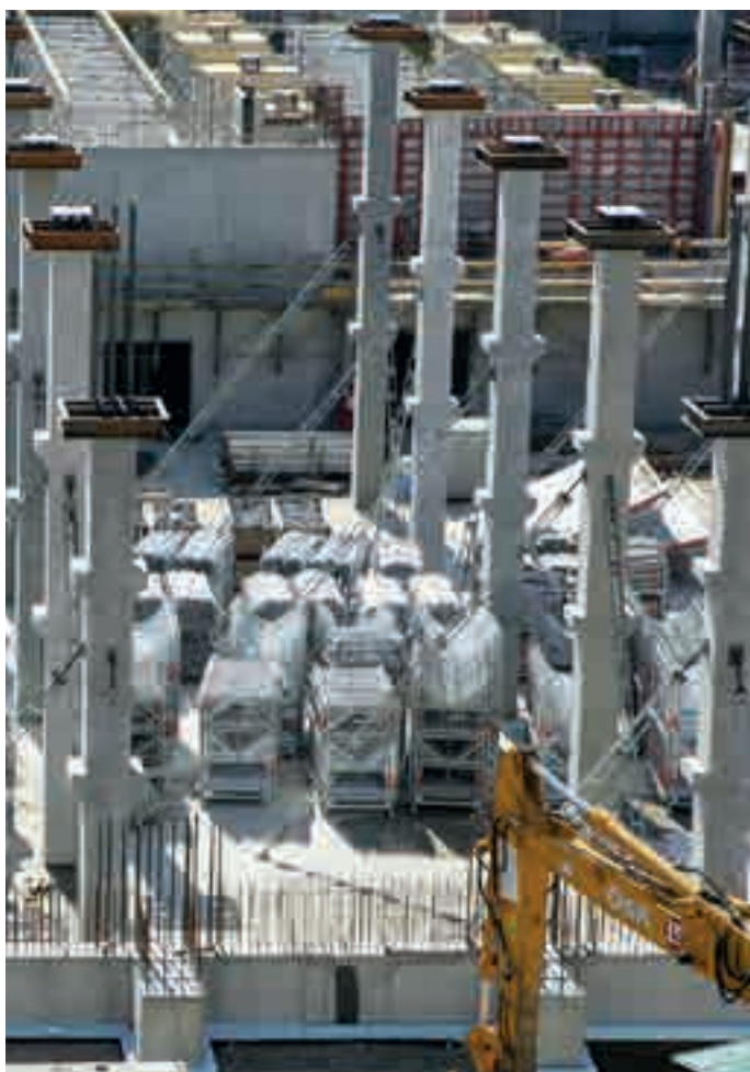
Filled pallets are lifted from the truck directly by a crane at the place of use.
