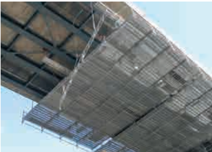
Suspended bridge underside scaffolding of lattice beams
