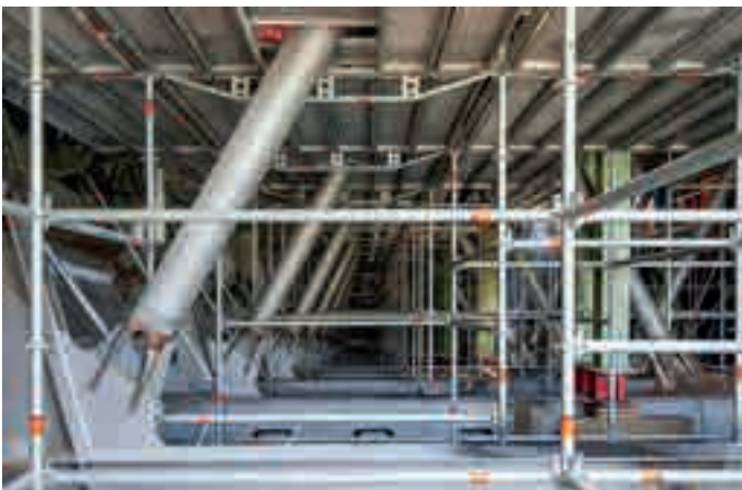
Work scaffolding inside box girders of bridge structure
