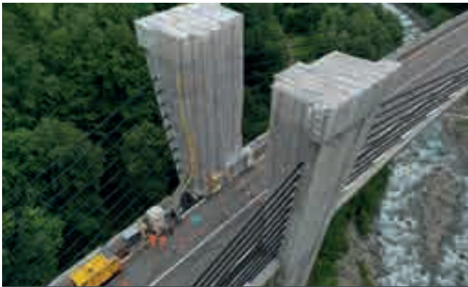
Cable-stayed bridge pylon covered by tarpaulins
