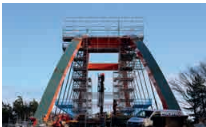
Self-supporting work scaffolding between the arches of an arched bridge with Allround FW System
