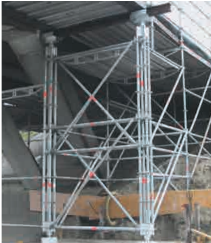
Heavy-duty support during bridge construction
