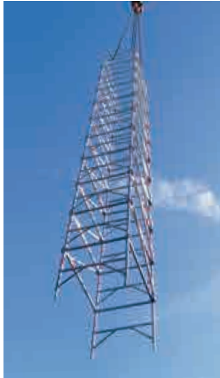
Crane movement of towers preassembled on the ground
