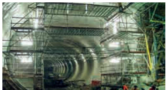
Mobile tunnel scaffolding running on rails with work platforms for safer working
