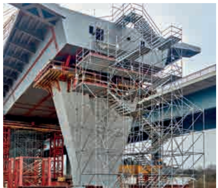
Site stairtower 200 for access to road surface, box girders and bridge bearings
