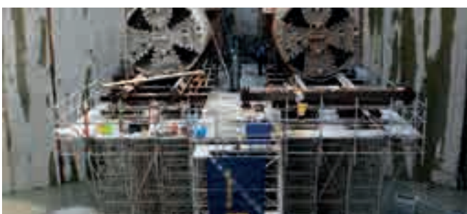
Drilling head support (shield cradle) on Allround Shoring TG 60 with integrated stairtower
