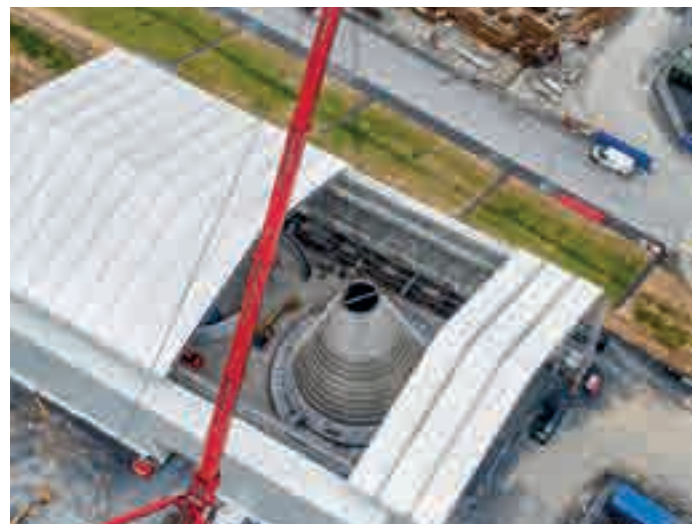
Opened mobile Keder Roof XL for lifting a funnel structure into place
