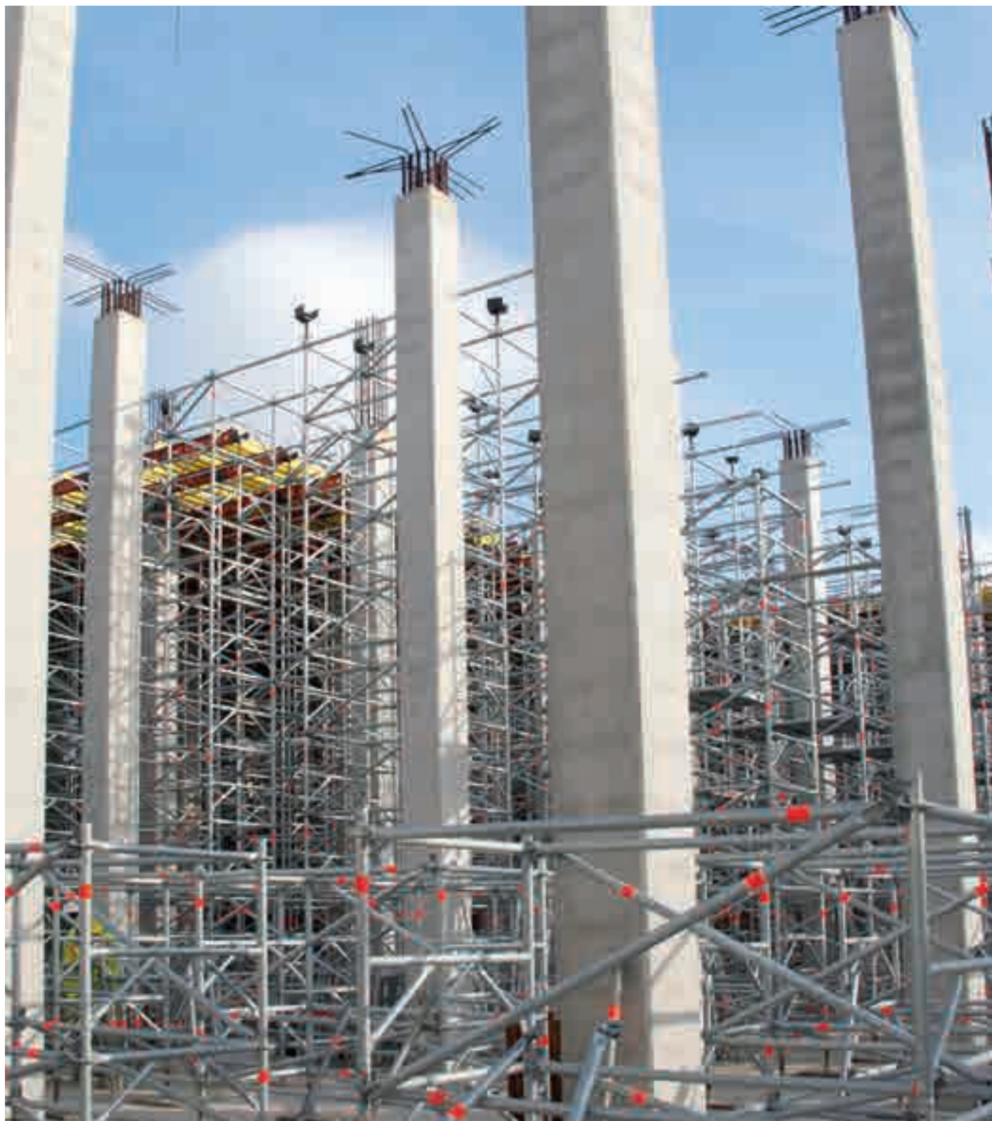
Connected shoring towers TG 60 during construction of a sewage plant – concrete pillars can simply be integrated into the shoring.
