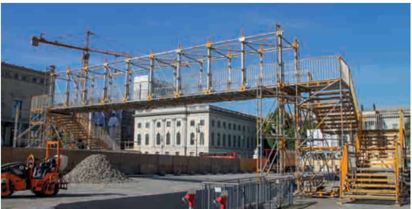
Temporary bridge over site with approx. 18 metre span to assist site logistics
