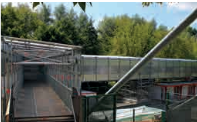
Temporary footbridge using Allround Bridging System with roofing and Protect enclosure
