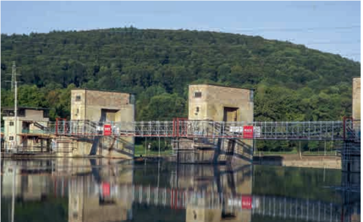
Temporary footbridge with a 2 x 34 metre span and an intermediate section with Allround Bridging System
