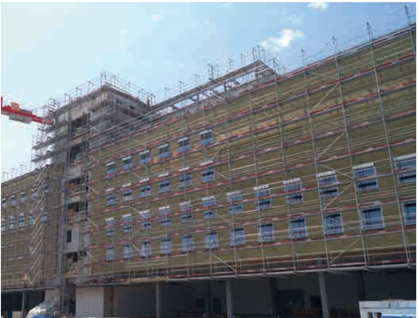
Facade work scaffolding of Layher SpeedyScaf resting on a projecting beam system to ensure continued vehicle access
