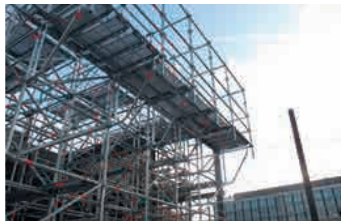
Integration of bracket-mounted walkways in shoring
