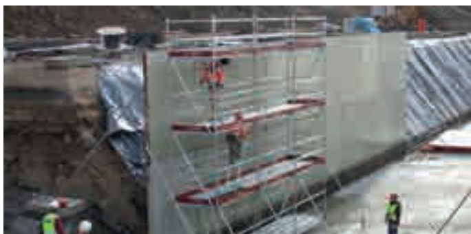
1.40 m wide reinforcing scaffolding with bracing
