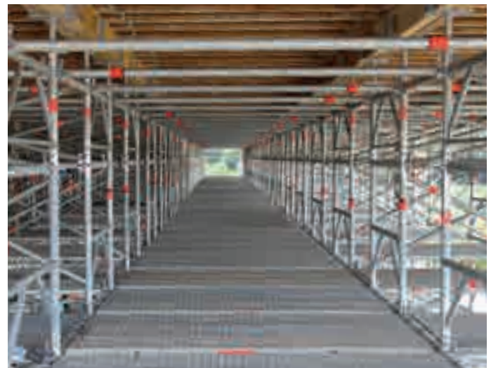
Integrated deck levels inside the shoring
