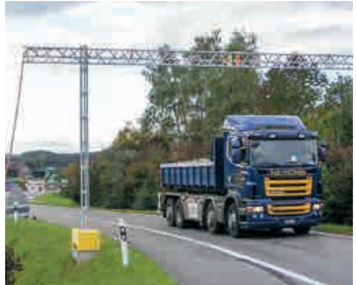
Cable bridge made of lattice beams and triangular supports including concrete ballast
