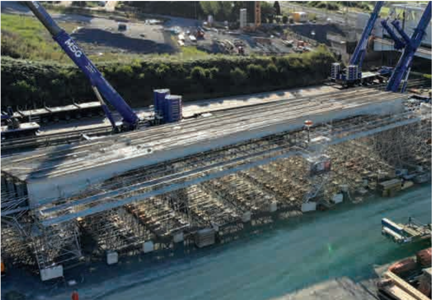
Shoring made from standard Allround components during construction of a new motorway bridge
