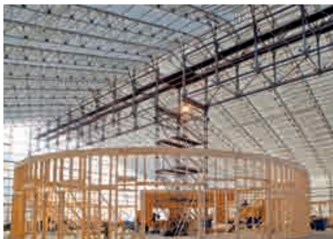
Keder Roof XL for wintertime timber construction work
