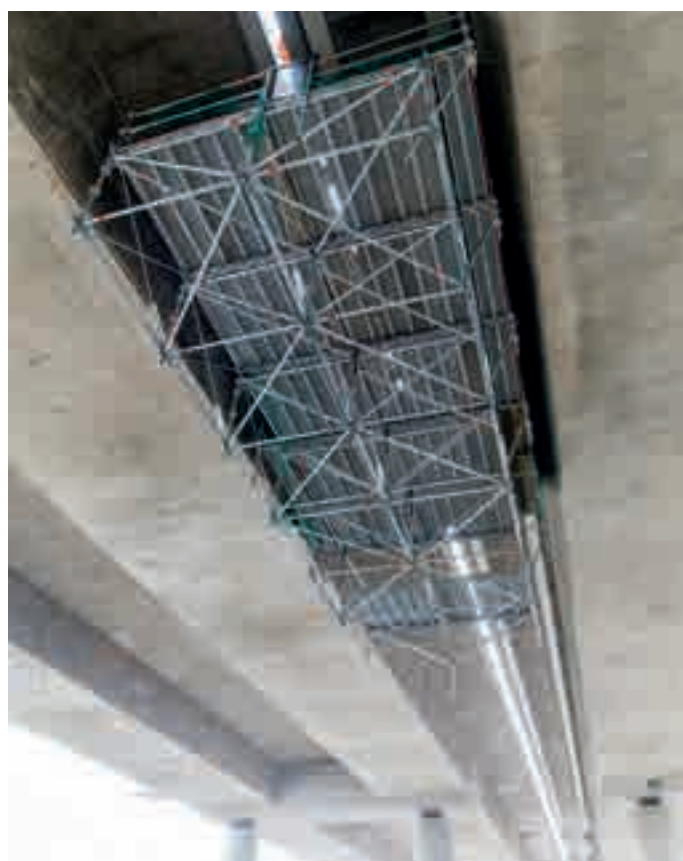
Mobile bridge underside scaffolding using Allround FW System and system decks
