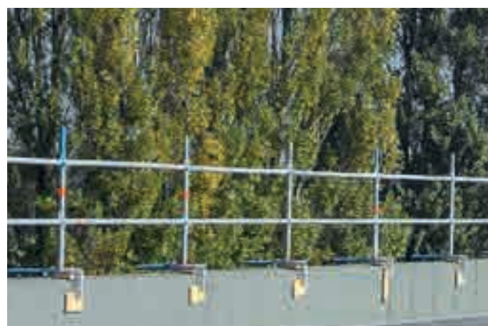
Use of a balustrade clamp on a flat roof with high fascia
