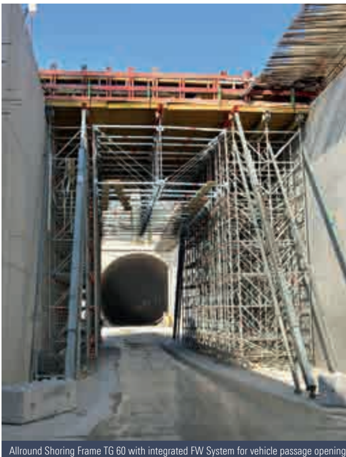
Frame combination for absorbing high loads of 22 tonnes per metre
