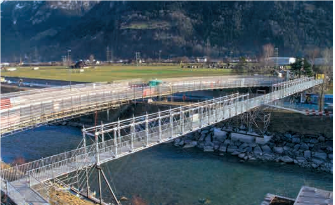
Temporary footbridge using Allround Bridging System with a span of 2 x 31 metres
