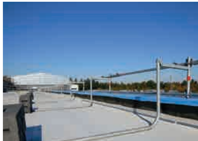
Flat roof side protection on a hall roof
