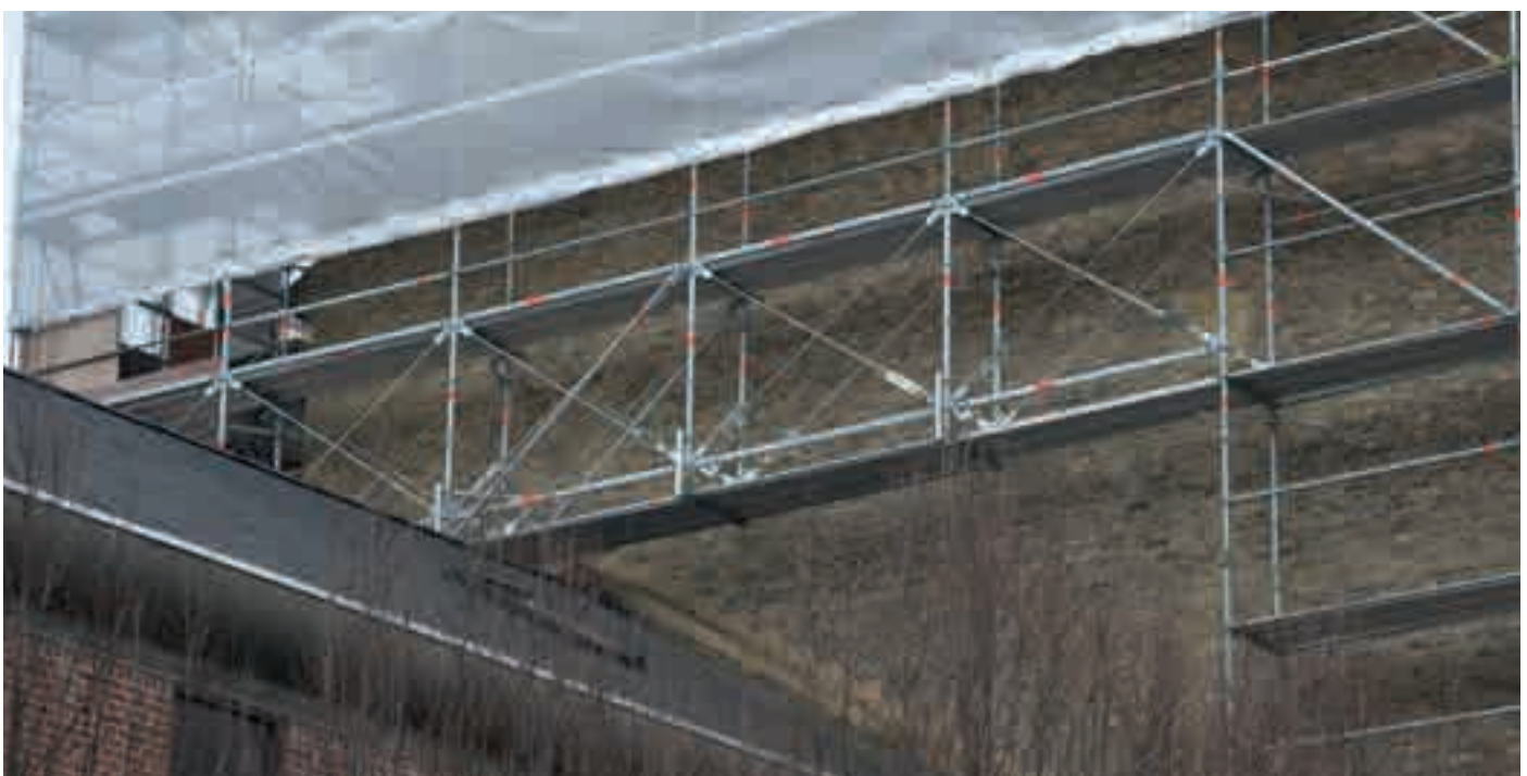
Bridging / supporting of work scaffolding using an external and non-loadable roof
