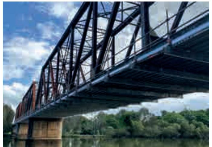
Suspended bridge underside scaffolding with protective wall on aluminium FlexBeam
