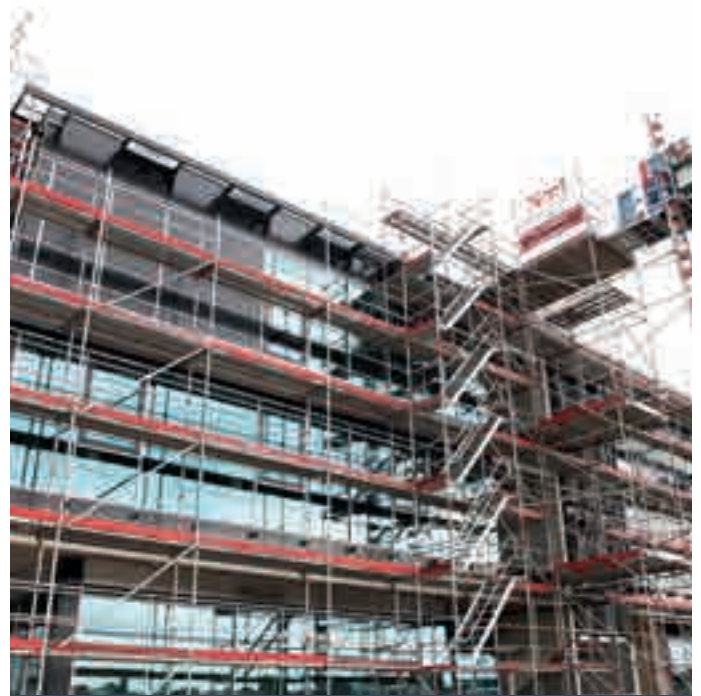
Allround work scaffolding with Allround Guardrail System
