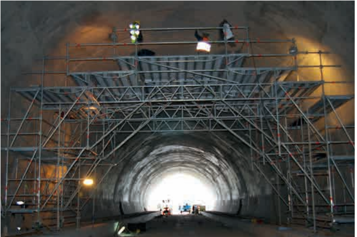
Mobile work scaffolding adapted to the tunnel geometry, with vehicle passage opening
