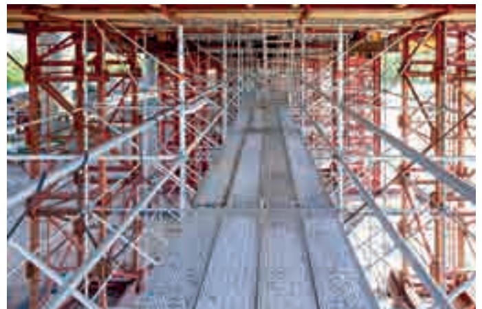
Work scaffolding inside box girders of bridge structure
