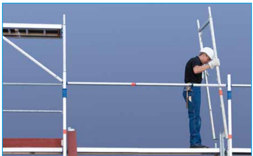
SpeedyScaf assembly with the Layher advance guardrail system
