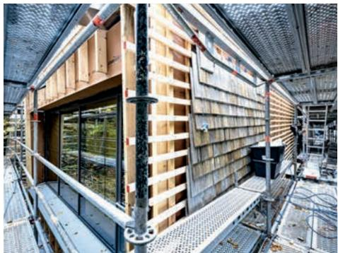
The entire complex was covered with pre-aged shingles to camouflage it as much as possible so that it blended into the surrounding forest. The Layher Allround Scaffolding and flexibly positioned platforms made the carpenters' work considerably easier.
