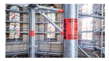
The top walk-on scaffold platform at 37.50 m in height, just underneath the main nave, allows the craftsmen and restoration experts to safely  $access\ their\ vertiginous\ workplace.$
