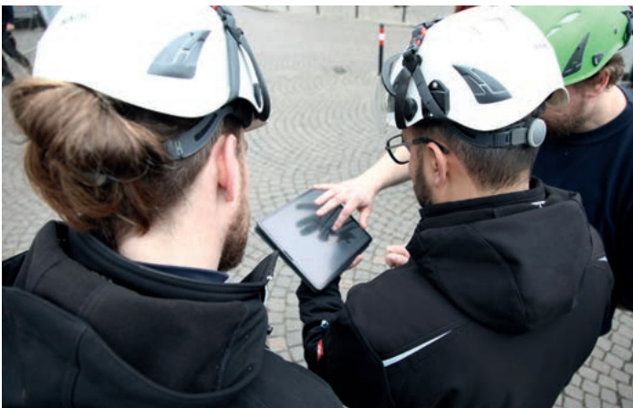
Digital planning documentation on site provides an overview.
