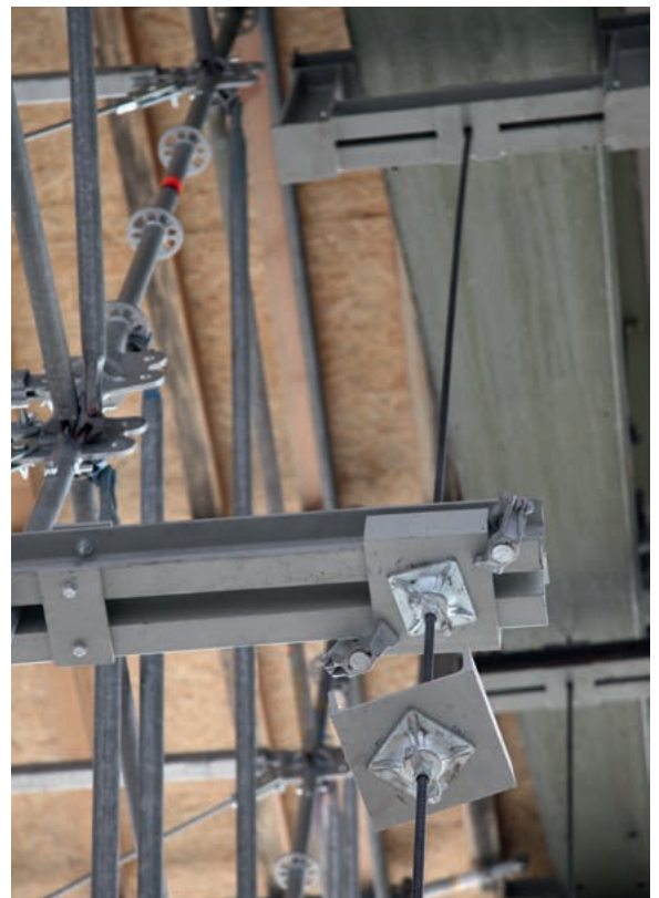
Brackets, metal rods and steel beams are used to suspend the Allround FW System.
