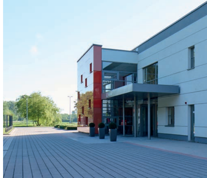
For many years, the Nietiedt headquarters in Wilhelmshaven has been an important partner for Layher far beyond northern Germany.
