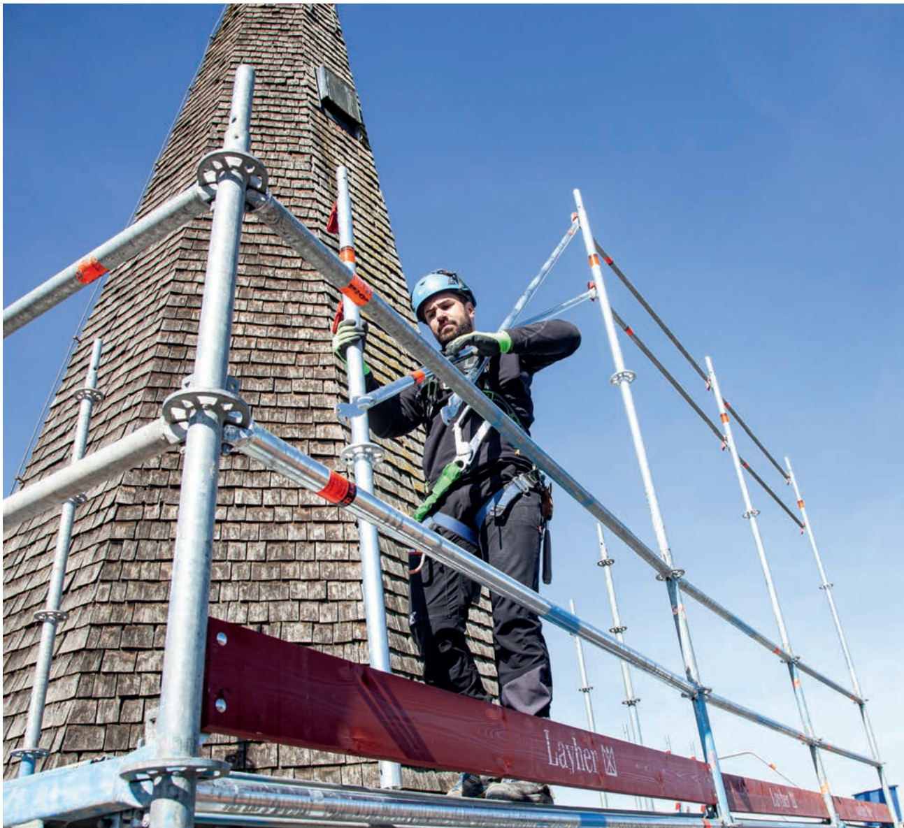
With the AGS System, assembly from a secured position is no problem.
