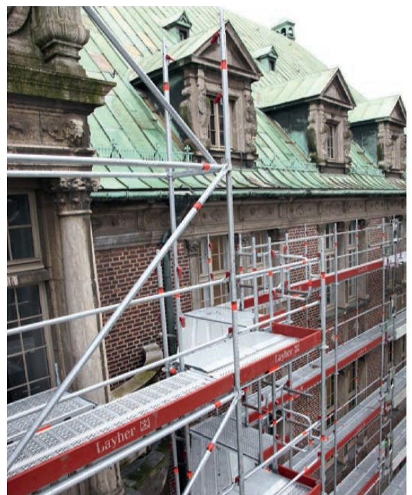
With U-steel decks and console brackets, scaffolding can be erected quickly and safely around large protrusions in the building envelope.
