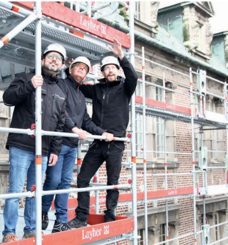
Wilh. Bädecker Gerüstbau GmbH Managing Director Malik Tharia (left), Layher Area Sales Manager Ingo Barge (centre) and Site Supervisor Lars Ukena (right)
