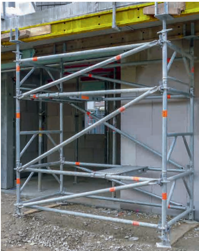
Stretched shoring tower TG 60 for supporting a balcony slab
