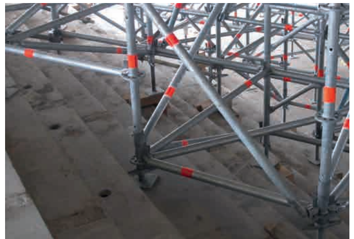
Adaptation of the shoring to stair flights with standard Allround material
