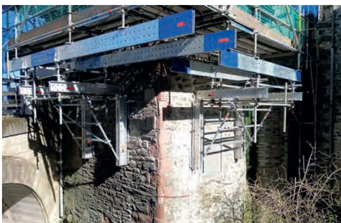
Suspended work scaffolding on a bridge pier of a stone bridge
