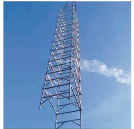
Crane movement of towers preassembled on the ground
