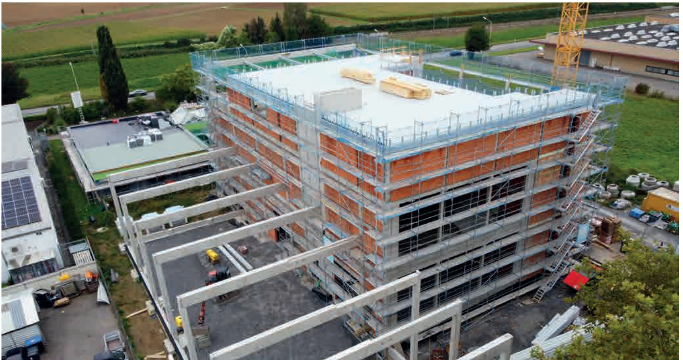
0.73 m wide Speedy work scaffolding with external platform stairway
