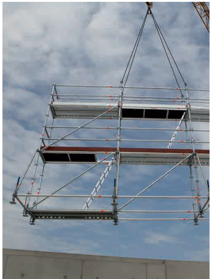
0.73 m wide reinforcing scaffolding with bracing during crane movement
