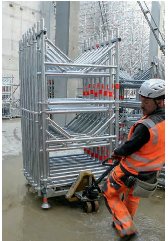
Filled TG 60 frame pallets can simply be moved on the construction site by a pallet truck.
