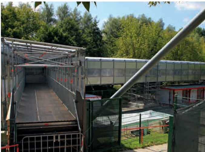
Temporary footbridge using Allround Bridging System with roofing and Protect enclosure
