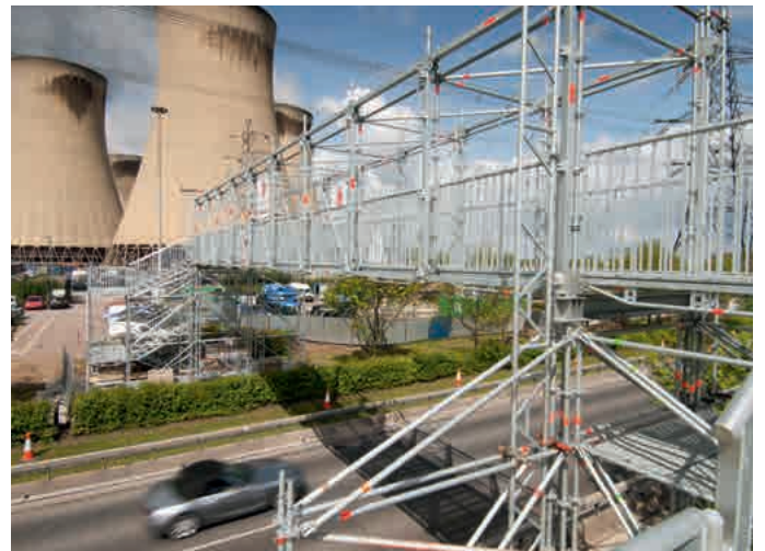
Temporary footbridge using Allround Bridging System with Stairtower 750 to assist site logistics
