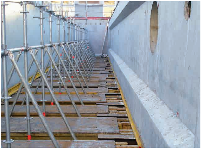
The variable system also permits support in the manufacture of tall and wall-like concrete beams cast in-situ, with semifinished ceiling slabs laid between them. Material optimisation by absorbing the ceiling loads using a latticework of Allround standard components between the shoring towers. No need for additional towers in the intermediate spaces.
