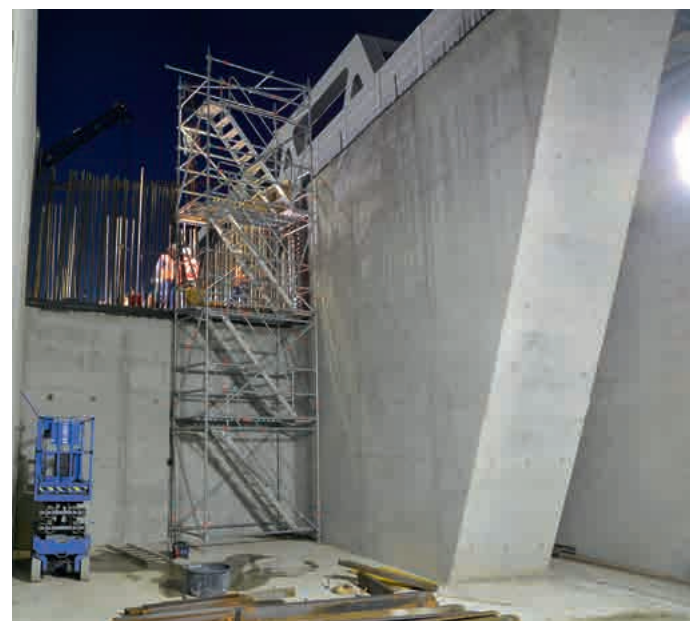
Access to bridge piers with Allround modular stairtower
