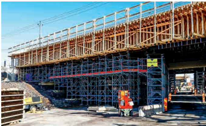
Shoring TG 60 with bracket-mounted walkways during construction of a road bridge
