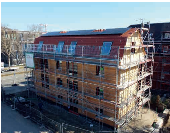
Speedy facade scaffolding with I-guardrails and integrated roof edge protection layer
