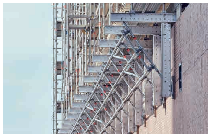
Suspended work scaffolding on TwixBeam consoles
