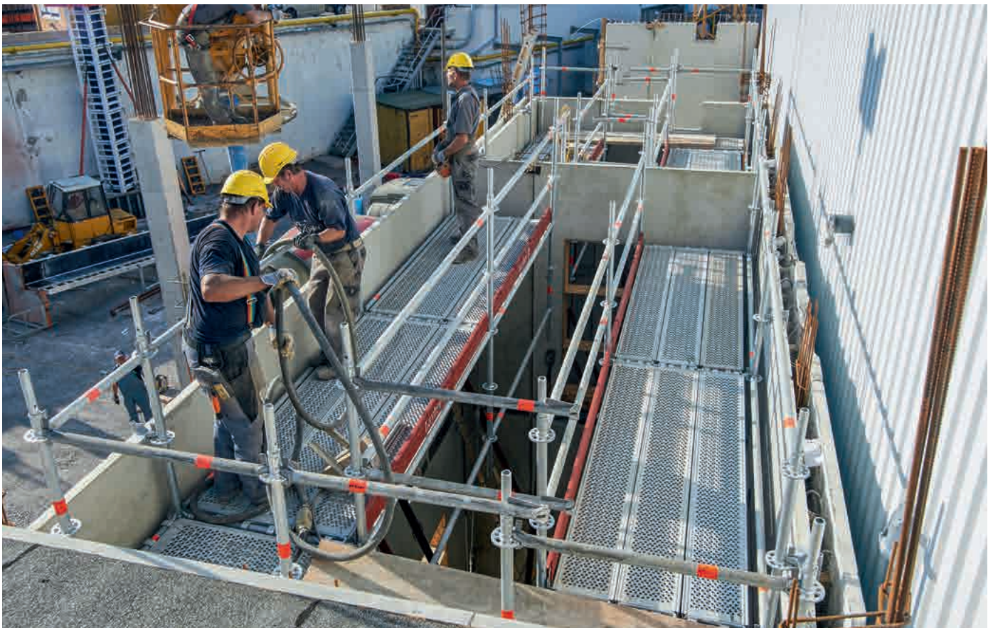
1.09 m wide concreting scaffolding with cavity wall bracket adapter
