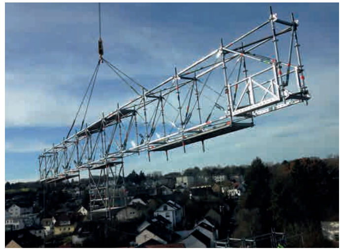
Crane movement of an FW System bridging structure
