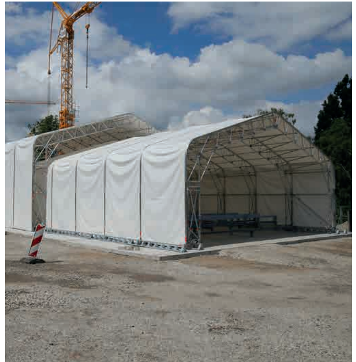
Interlocking Keder Halls for the production of concrete parts
