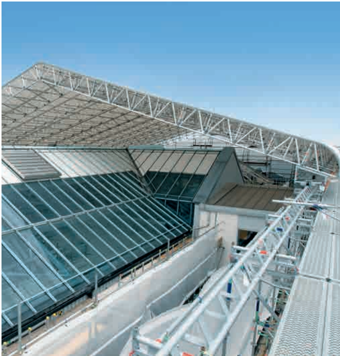
Mobile Keder Roof XL during roof work at a shopping centre
