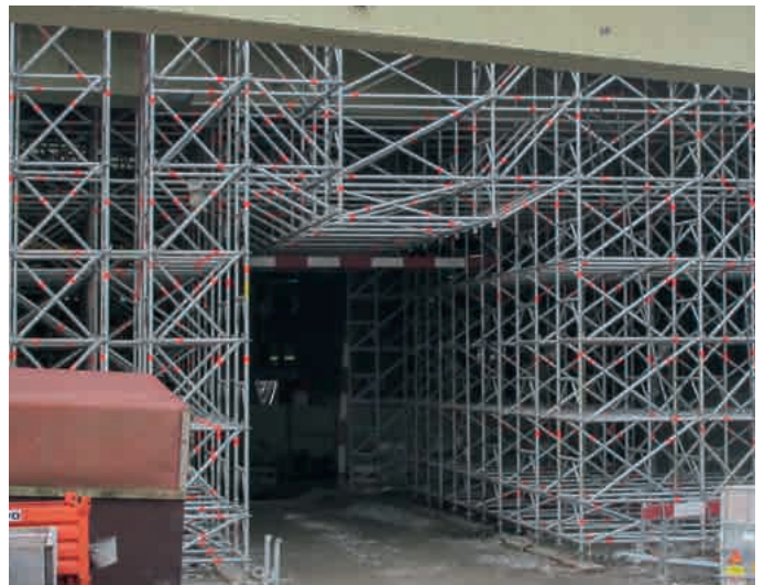
Vehicle passage opening thanks to the use of Allround standard material
