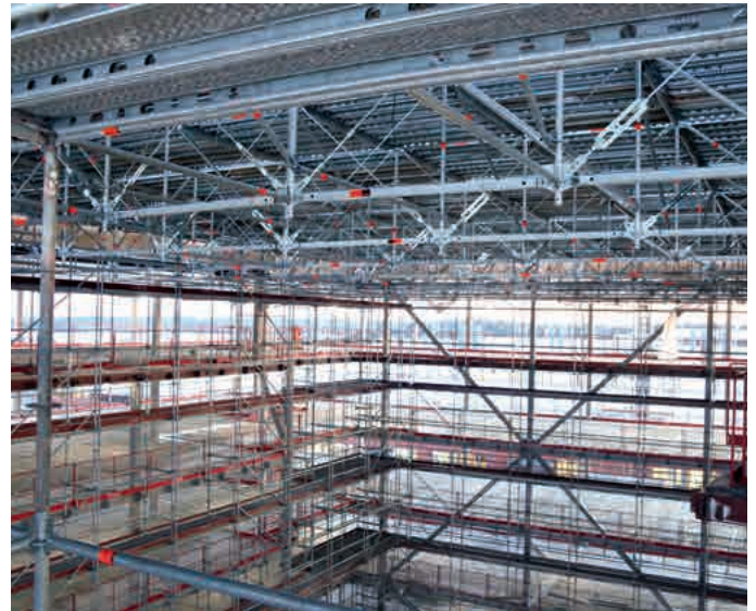
Self-supporting birdcage scaffolding in a shopping centre
