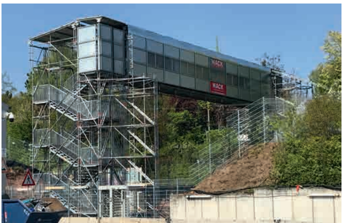
Temporary footbridge with Protect enclosure and cassette roof
