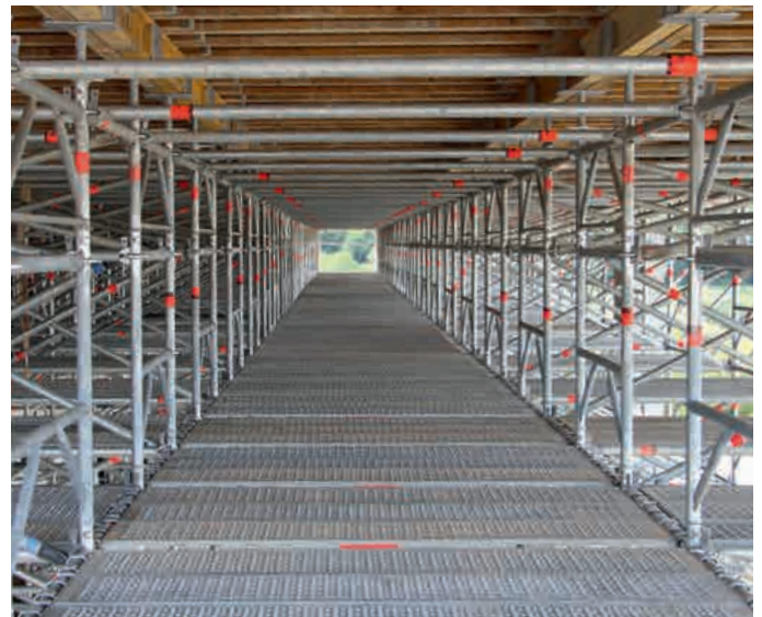
Integrated deck levels inside the shoring
