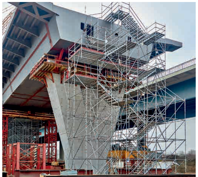
Site stairtower 200 for access to road surface, box girders and bridge bearings
