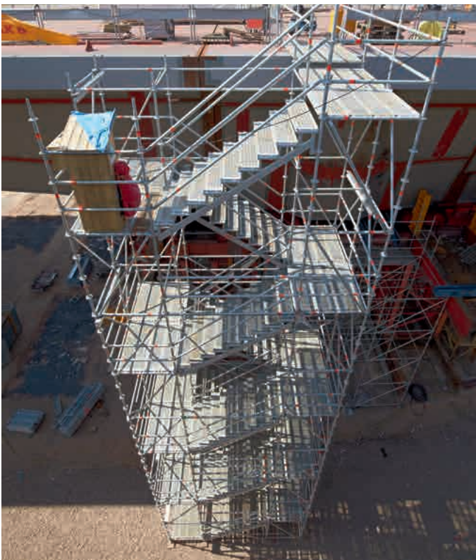
Site stairtower 200 for access to road surface
