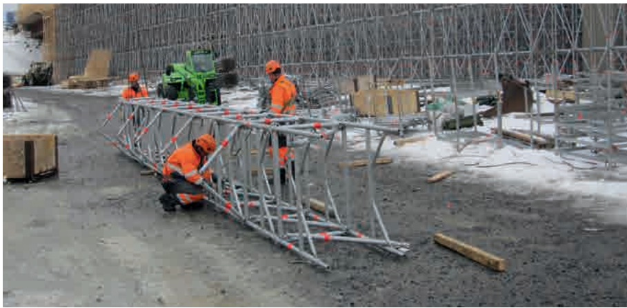
Assembly of a TG 60 Shoring Tower on the ground
