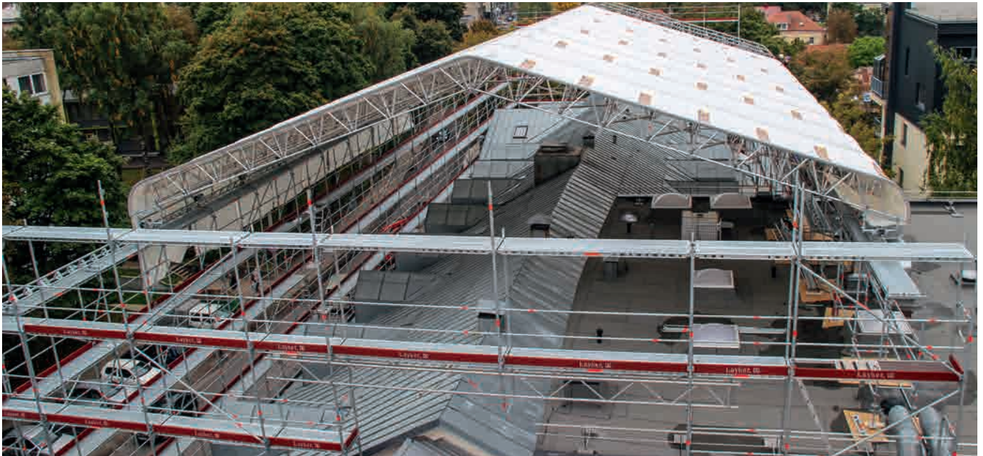
Mobile Keder Roof XL on SpeedyScaf during roof work on an office building
