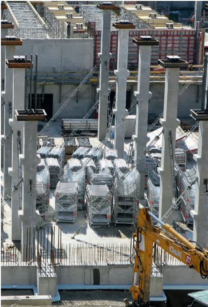
Filled pallets are lifted from the truck directly by a crane at the place of use.
