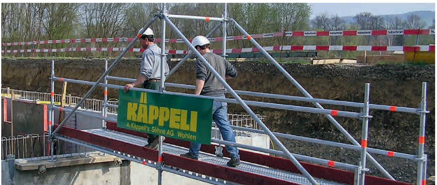
Trench bridge of two Allround Scaffolding bays
