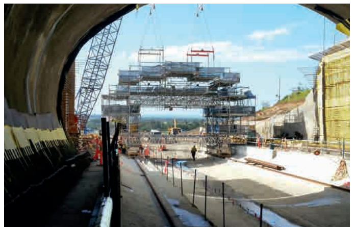
Previous emplacement of a preassembled mobile tunnel scaffolding by crane
