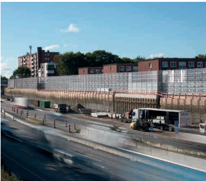
Noise control wall for reducing traffic noise
