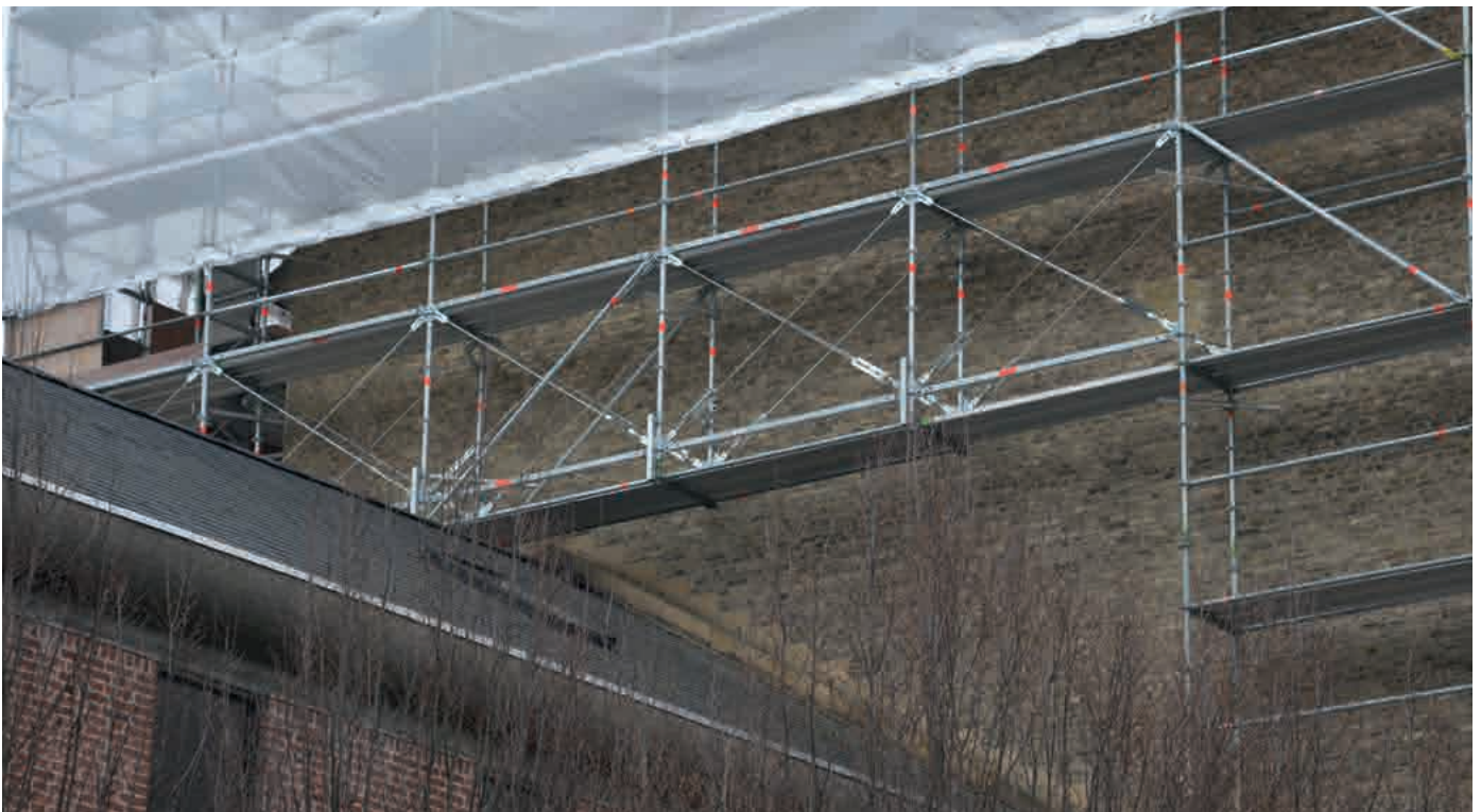
Bridging / supporting of work scaffolding using an external and non-loadable roof
