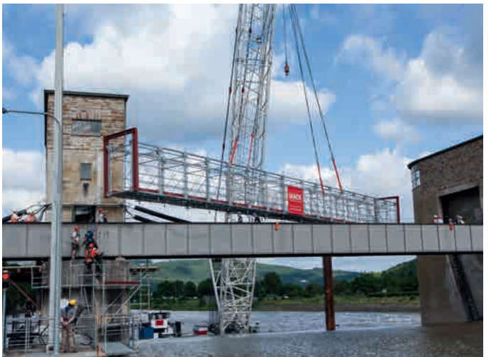
Lifting the temporary bridge into place using a floating crane
