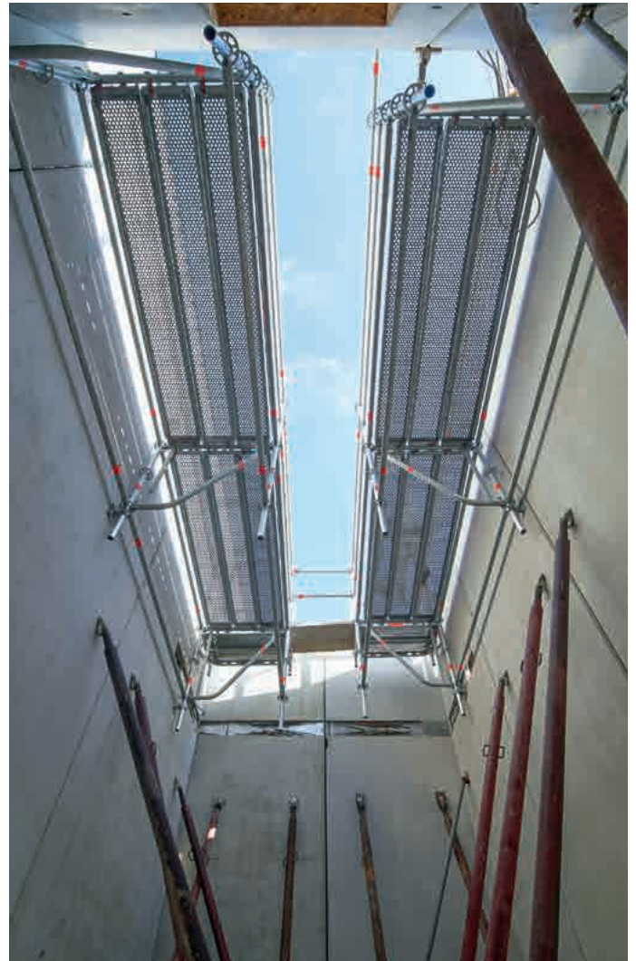
The space underneath the scaffolding remains free for the push-pull props.
