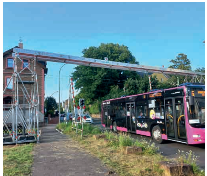
Cable bridge of FlexBeams on Allround support towers
