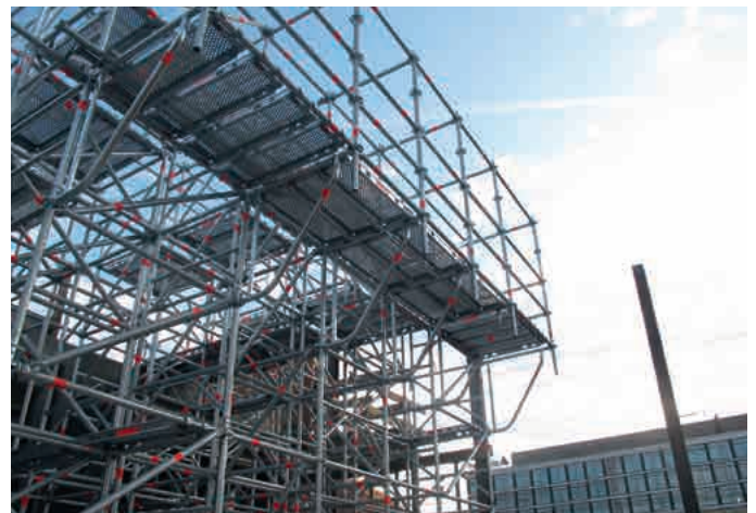
Integration of bracket-mounted walkways in shoring
