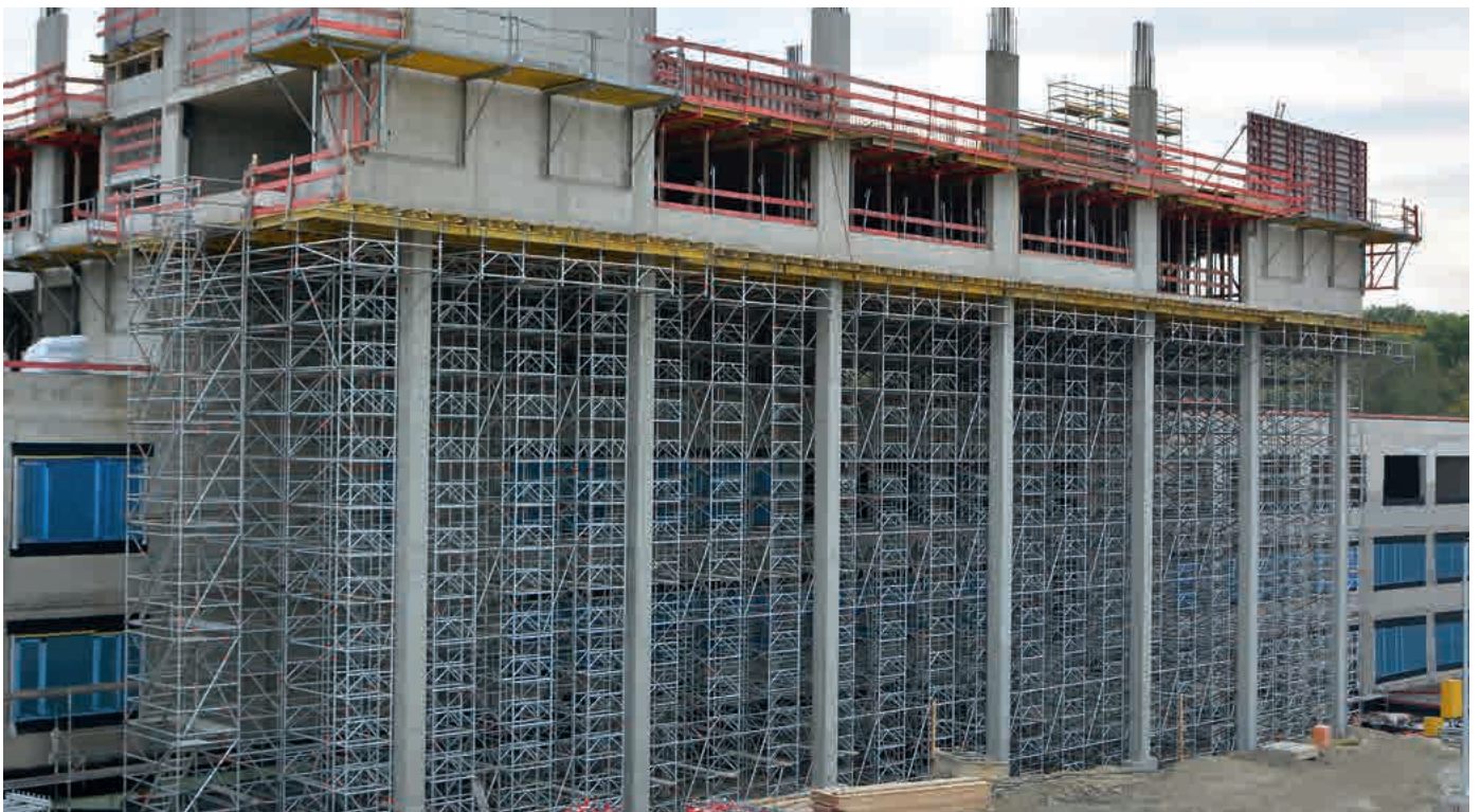
Combination of Allround Shoring Towers TG 60 for concreting of a projection — fast and convenient site access with Allround modular stairtower
