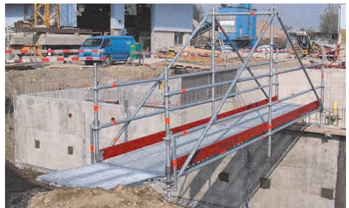
Trench bridge of two Allround Scaffolding bays
