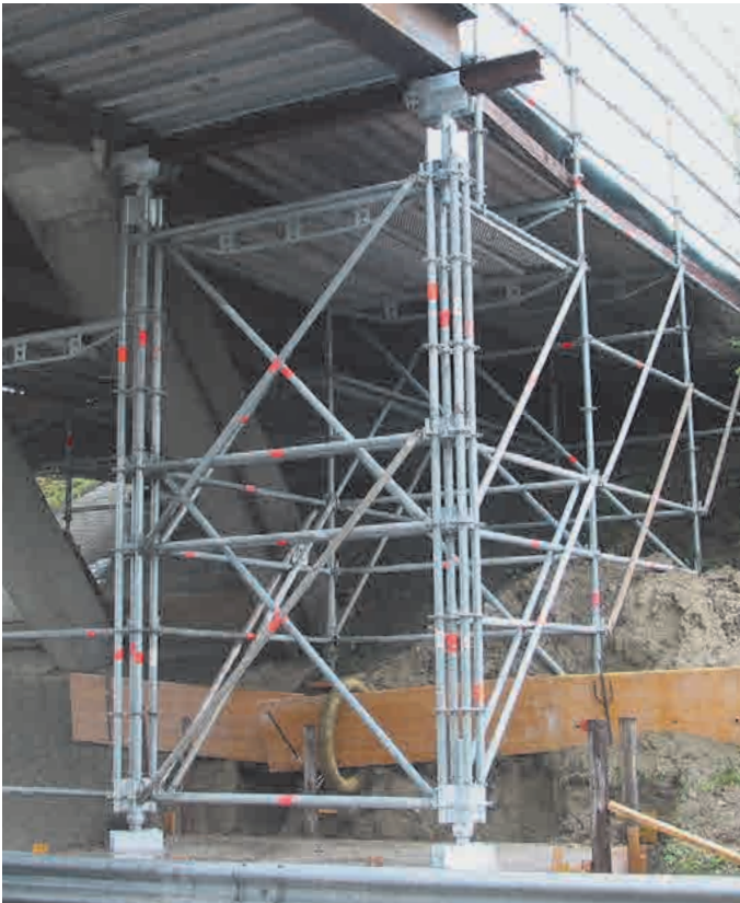
Heavy-duty support during bridge construction
