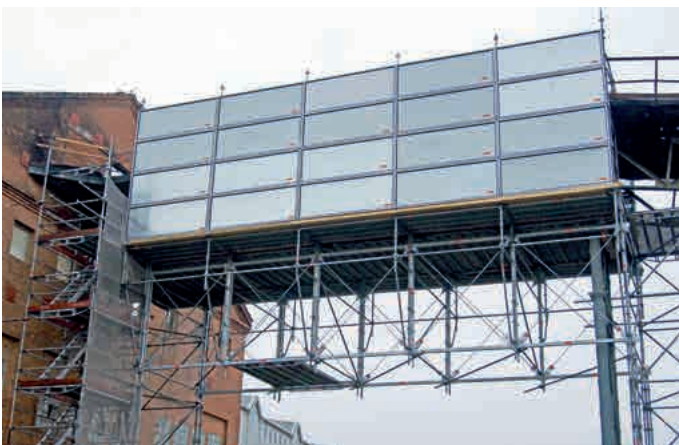
Work scaffolding covered using the Protect System on a pipeline bridge for fire damage repair
