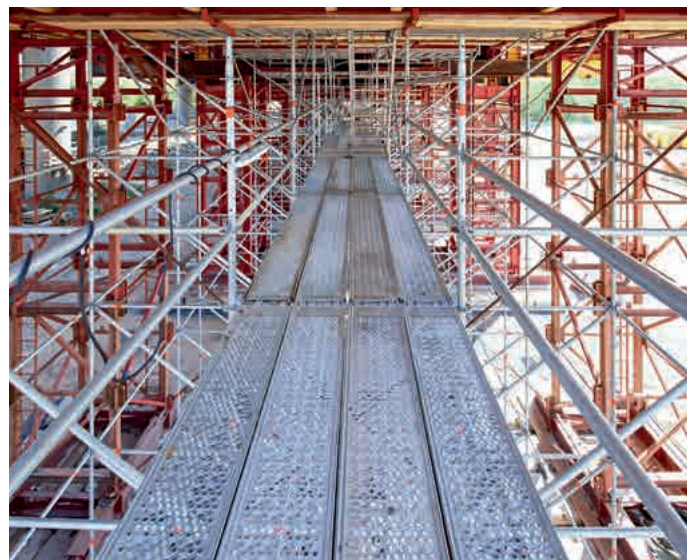
Work scaffolding inside box girders of bridge structure
