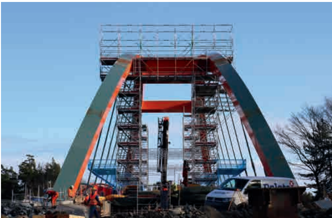
Self-supporting work scaffolding between the arches of an arched bridge with Allround FW System
