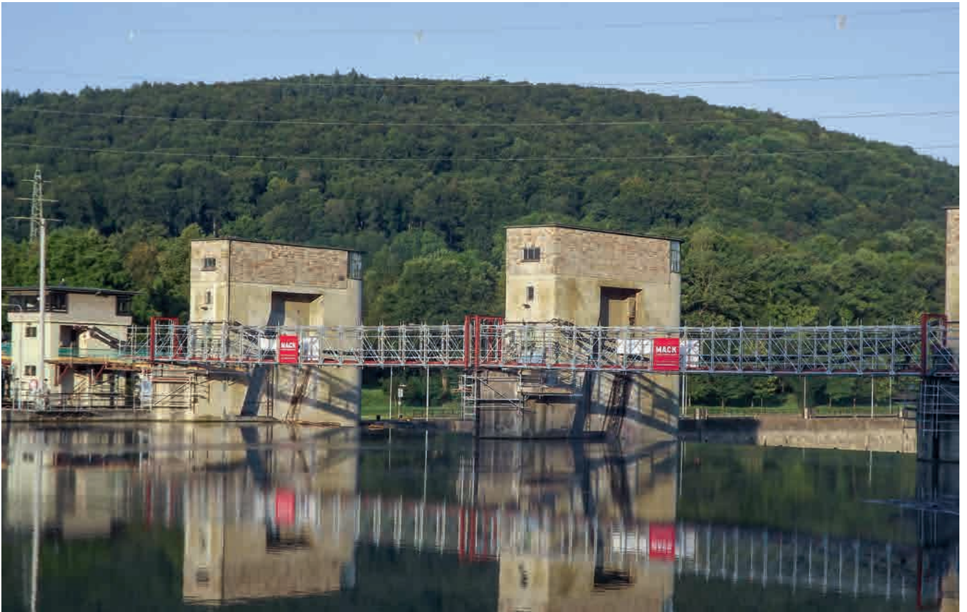
Temporary footbridge with a 2x 34 metre span and an intermediate section with Allround Bridging System
