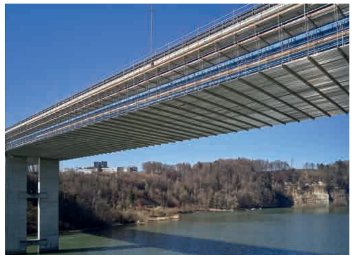
Approx. 7000 m 2 -sized bridge underside scaffolding with FlexBeam at a steel composite bridge
