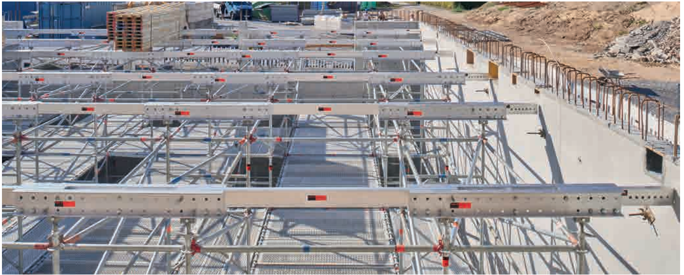
TwixBeam aluminium beam as a system main beam – the insertion beam serves as a connection between the TwixBeam beams and for adaptation to the edge area of the ceiling formwork.
