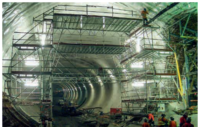
Mobile tunnel scaffolding running on rails with work platforms for safer working
