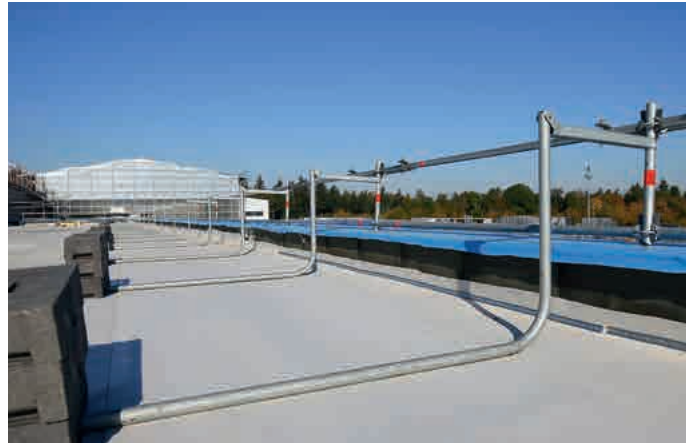
Flat roof side protection on a hall roof
