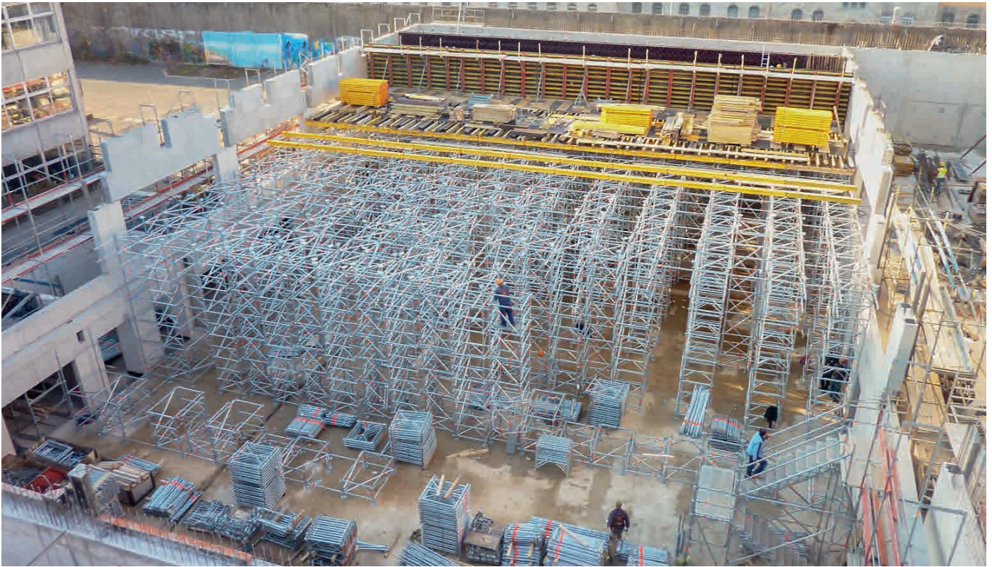
The variable system also permits support in the manufacture of tall and wall-like concrete beams cast in-situ, with semifinished ceiling slabs laid between them. Material optimisation by absorbing the ceiling loads using a latticework of Allround standard components between the shoring towers. No need for additional towers in the intermediate spaces.
