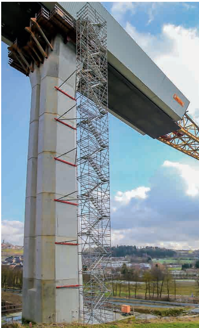
Access to bridge piers with Allround modular stairtower
