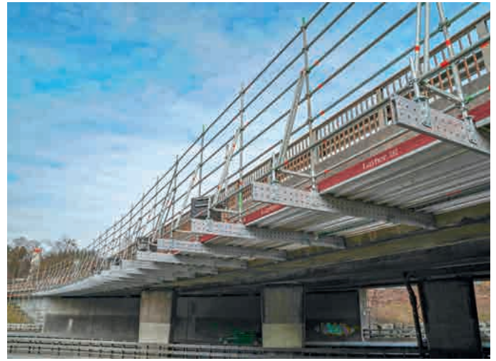
Bridge underside scaffolding with protective wall made from Aluminium FlexBeam
