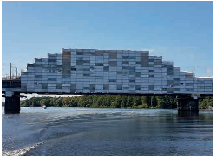
Bridge work scaffolding enclosed with cassette roof and Protect System
