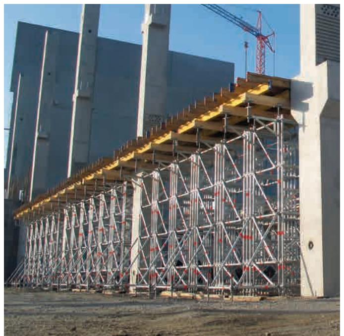
Vehicle passage opening thanks to the use of Allround standard material
