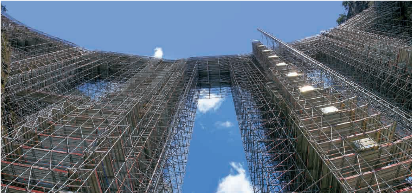
Free-standing work scaffolding on stone arched bridge
