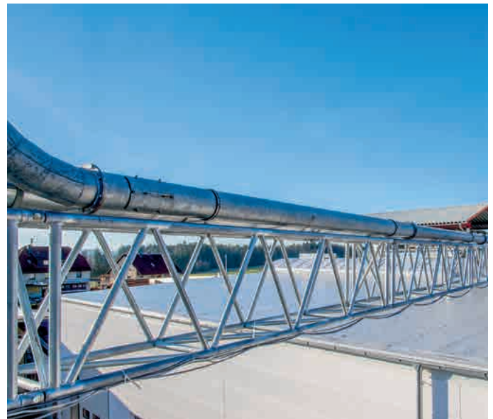
Pipeline bridge using steel trusses
