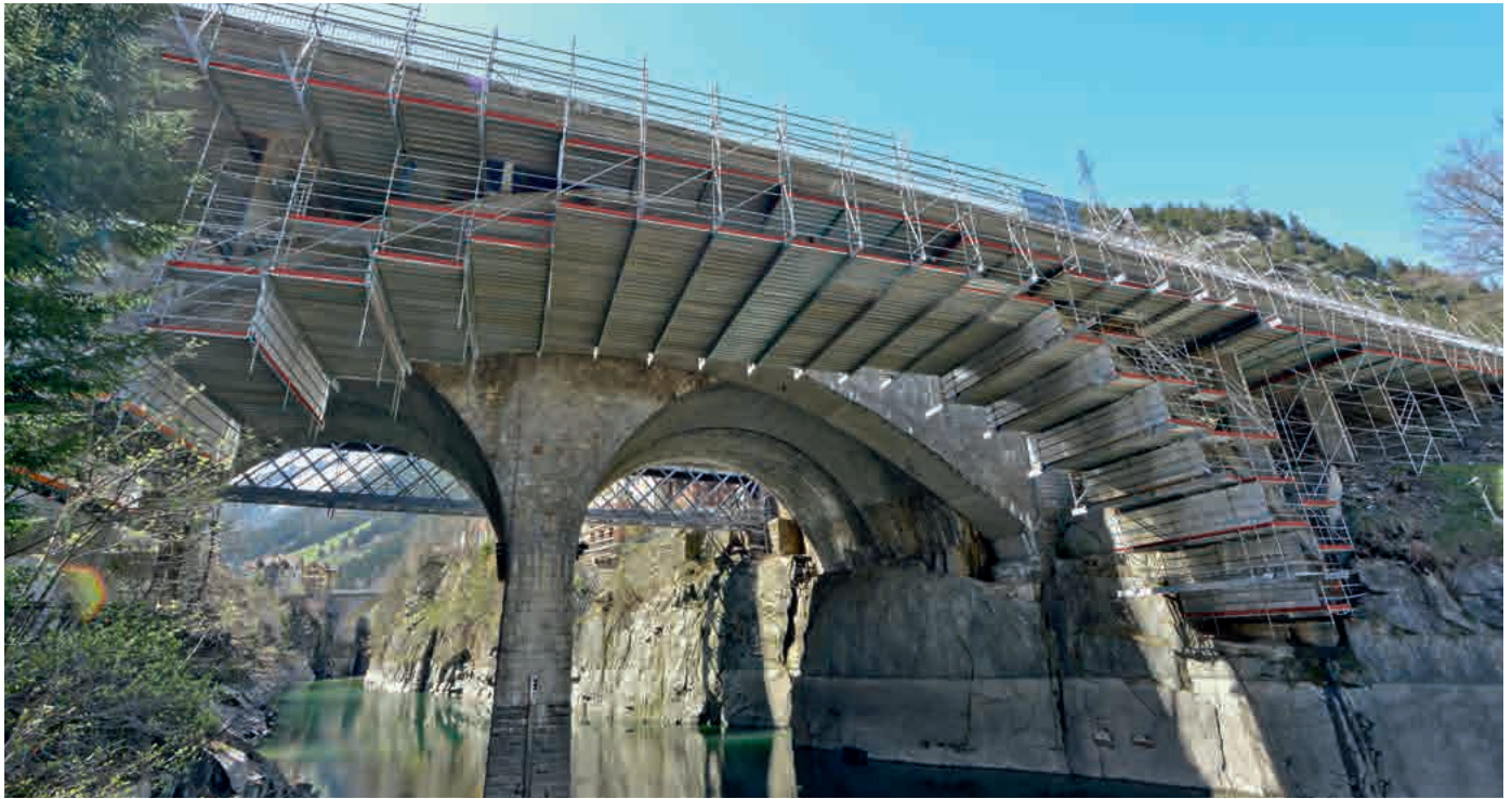
Bridge underside scaffolding with two levels made from Aluminium FlexBeam at a viaduct
