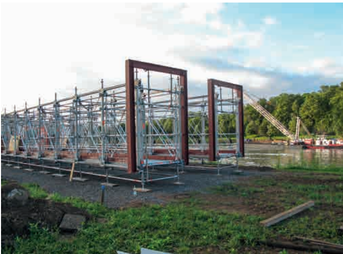
Preassembled bridges for subsequent lifting into place by crane
