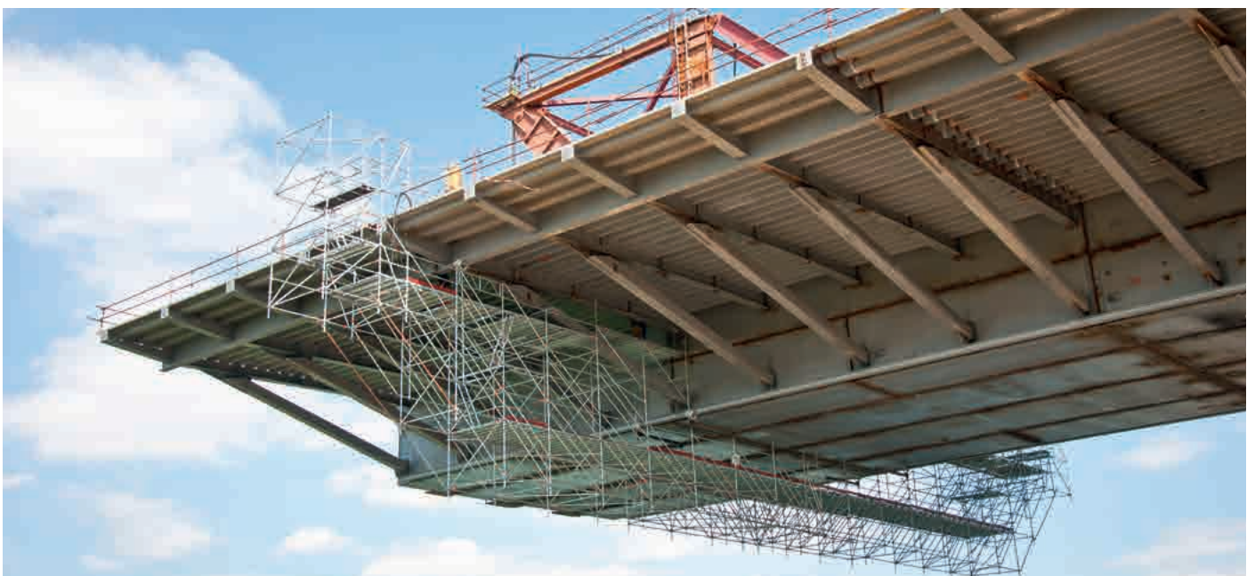
Mobile bridge underside scaffolding made of Allround system components
