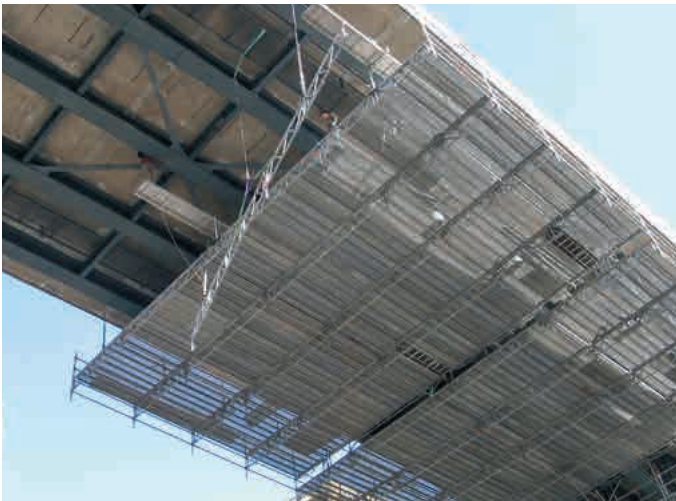
Suspended bridge underside scaffolding of lattice beams
