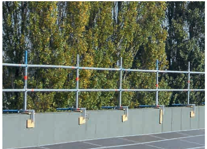
Use of a balustrade clamp on a flat roof with high fascia
