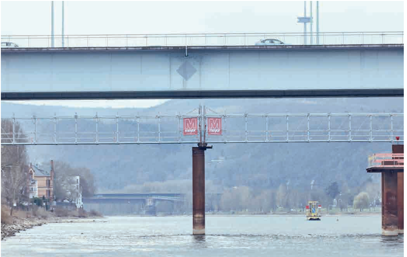
Temporary footbridge using Allround Bridging System with a span of 2 x 31 metres
