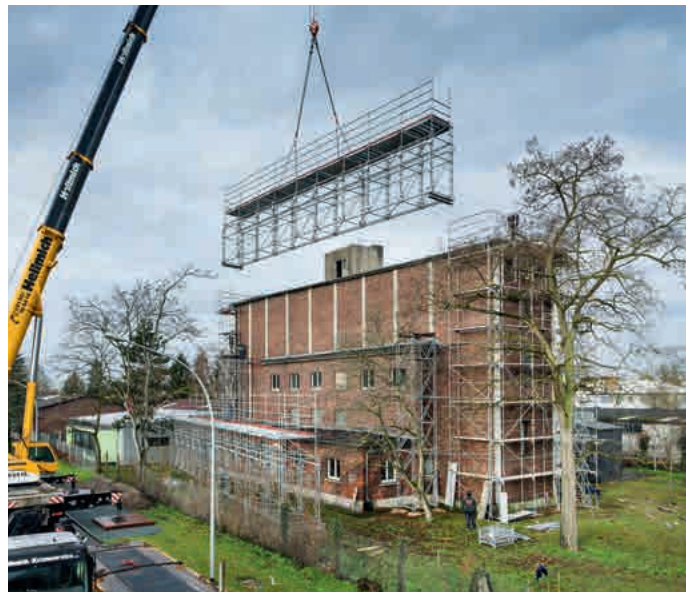
Bridging / supporting of work scaffolding using an external and non-loadable roof
