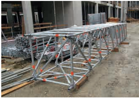
Preassembly of TG 60 Shoring Tower on the ground
