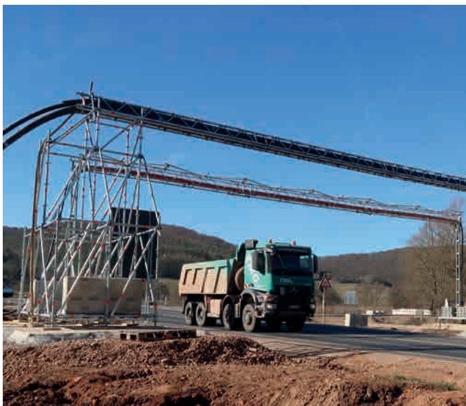
Cable bridge of lattice girders and tri-struts including concrete ballasting
