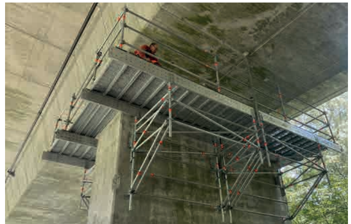
Work scaffolding on bridge pier with FlexBeam on Allround wall bracket
