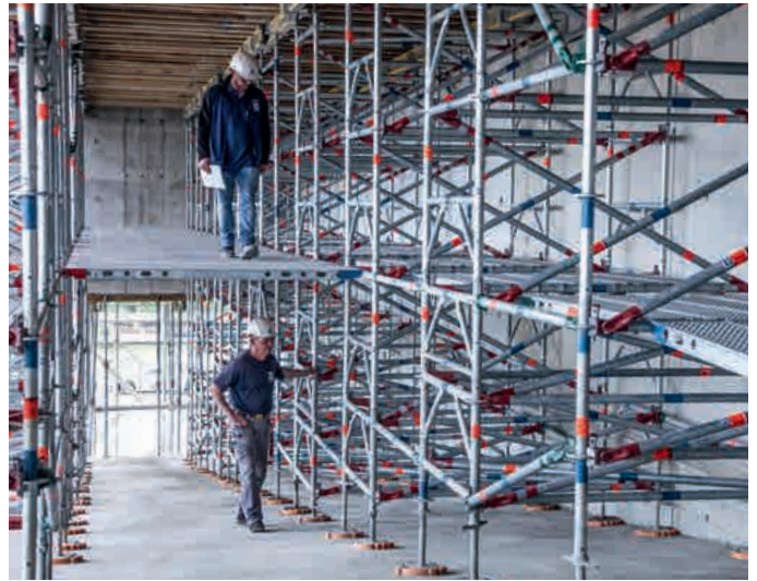
Integrated deck levels inside the shoring, and shoring adapted to the slope of the ground using equalising plates
