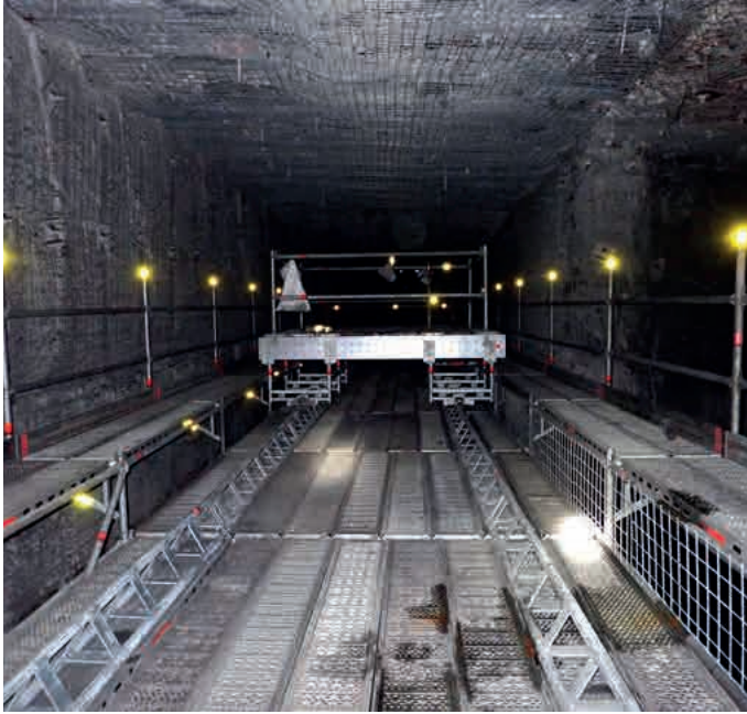
Mobile tunnel drilling podest, Australia
