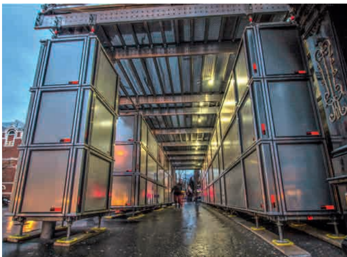
Work scaffolding with pedestrian tunnel with FlexBeam and Protect enclosure
